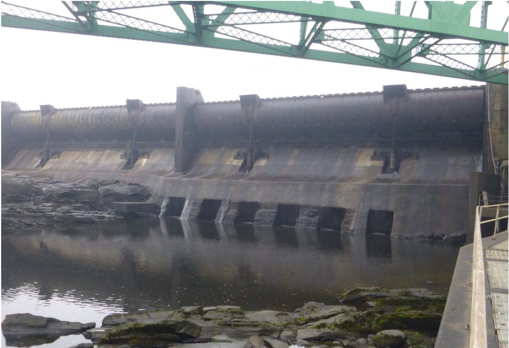
**Figure 5.4-2: Spillway Gate ‘Teeth’ That Were Not Represented in the Spillway CFD Model**
