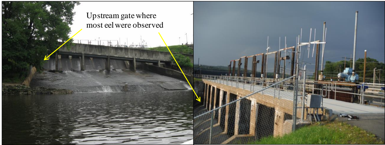
Photo 1. Locations where eel were observed at the Cabot Emergency Spillway.
