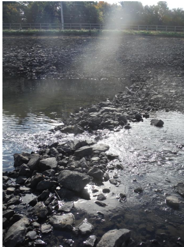
Photo 10. Riprap "weir" spanning canal bed in Zone 6. Note upstream direction of flow (Day 2).
