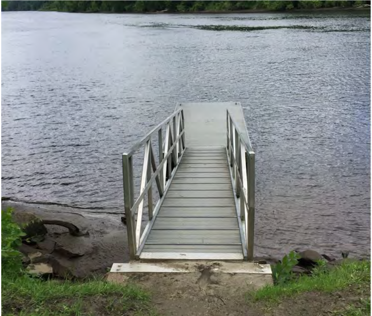
Figure 4.2.3-1 Munn's Ferry Boat Camping Recreation Area Floating Boat Dock
