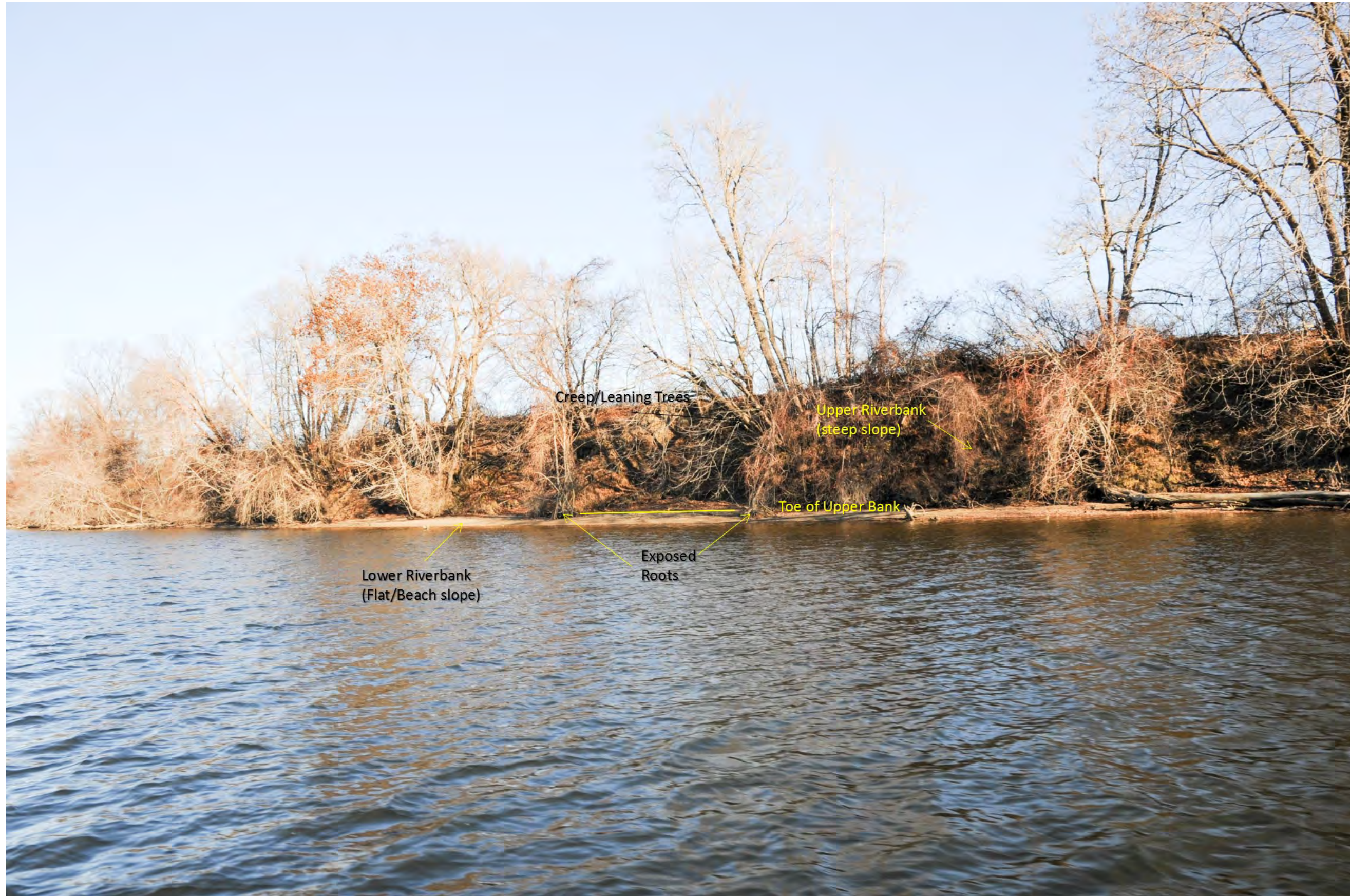
Photo ID 650 (left, U/S portion of segment)
