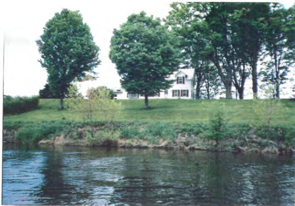
NUSCO installed 330 ft of riprap at this site across from Munn's Ferry in 1977 - May 22, 1990.
