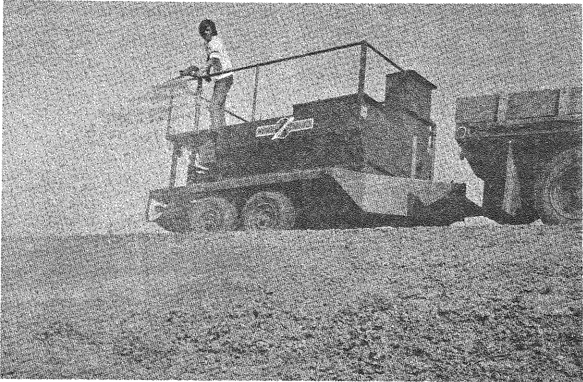
Figure 83. Mechanical broadcaster spreading mulch on top of stream bank.
