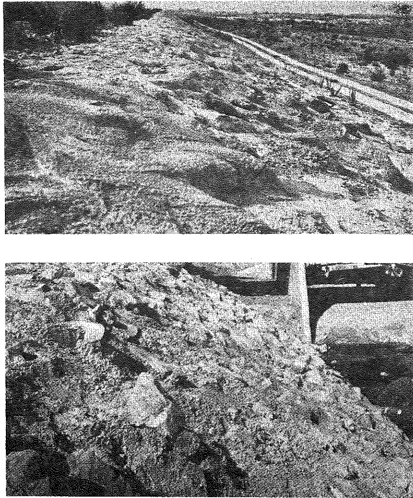
Figure 87. Examples of rough textured grouted-rock protection (California Division of Highways, 1960).
