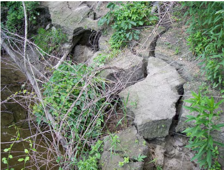
Erosion at toe of bank (jpeg.143)
