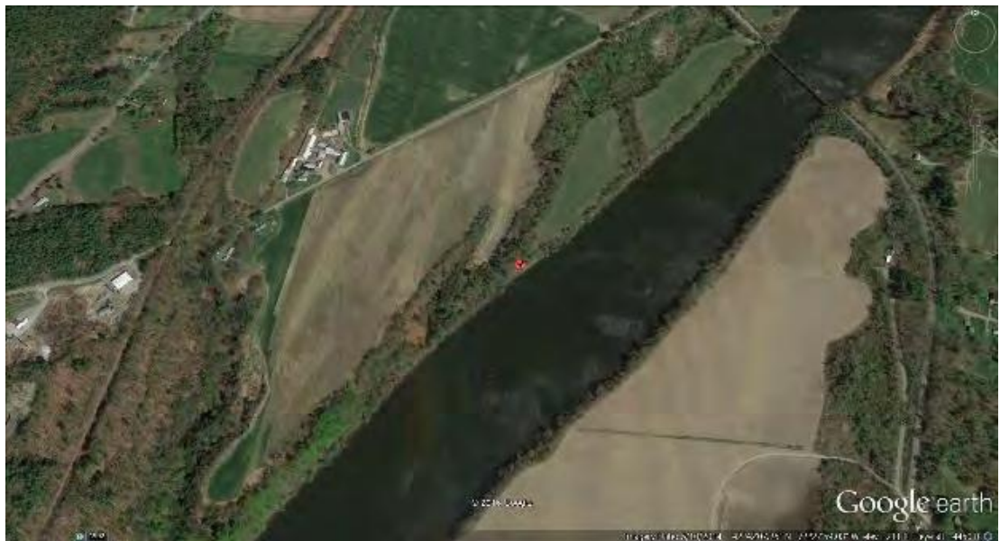
Figure 5.5.4-5: Irrigation pumping from the Connecticut River and Location on Google Earth, Photo 255
