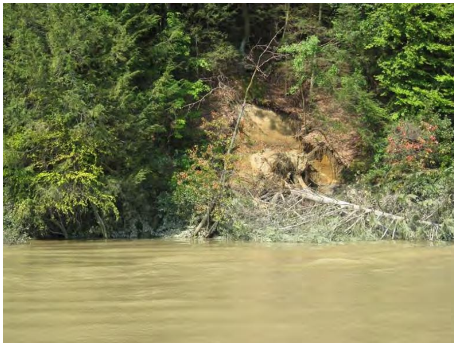
Figure 5.5.5.5-16 Erosion Due to High Flow in 2011
