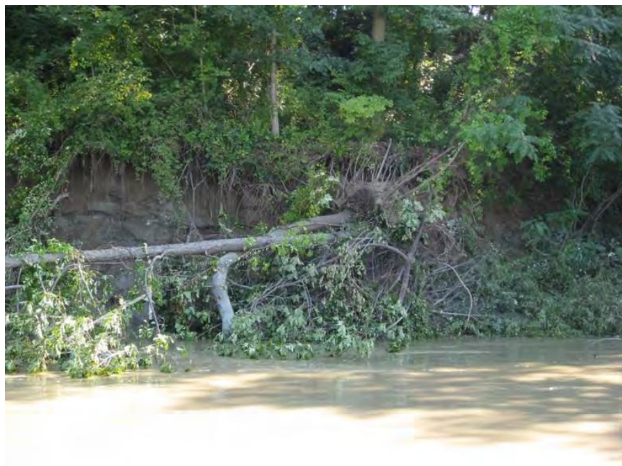
Figure 5.5.5.5-17 Erosion Due to High Flow in 2011
