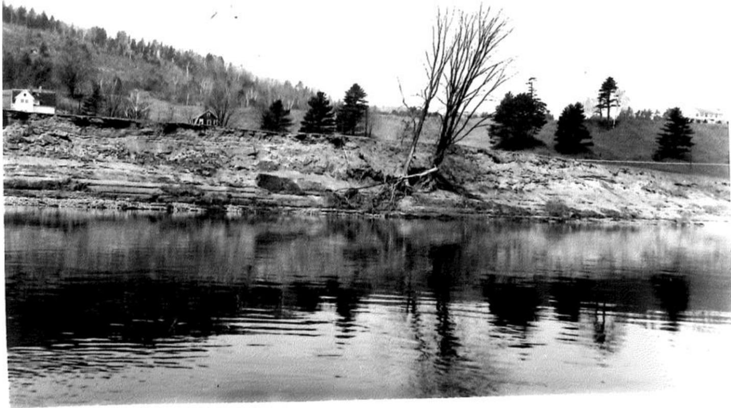
Figure 5.5.5-18 Erosion in 1946 Due to Ice (TransCanada)
