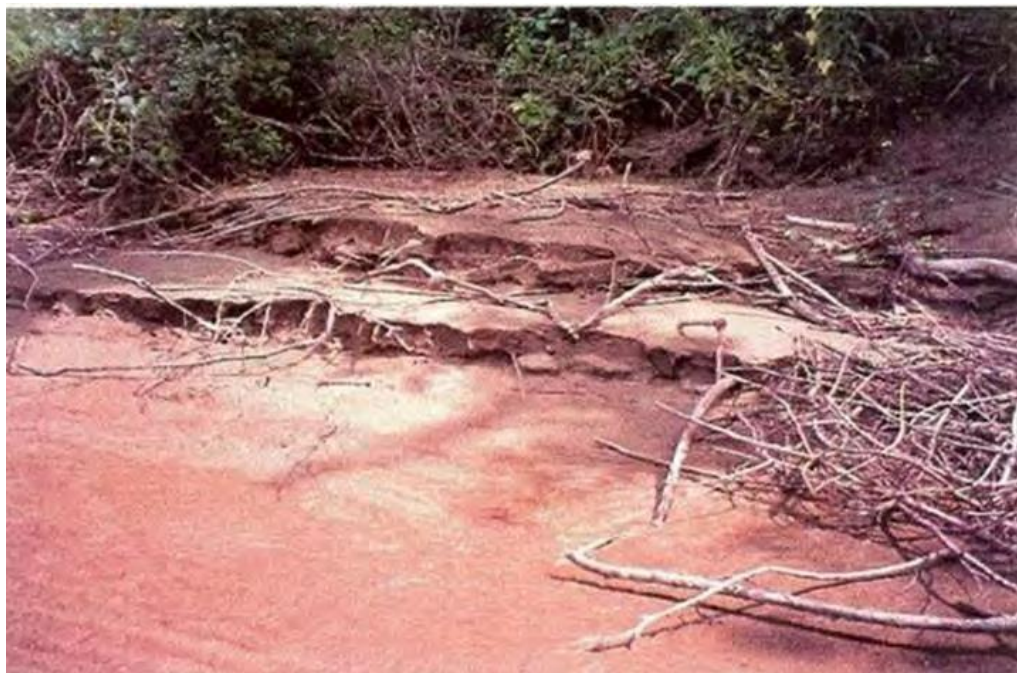
Figure 5.5.3-3: Notching Due to Boat Waves
