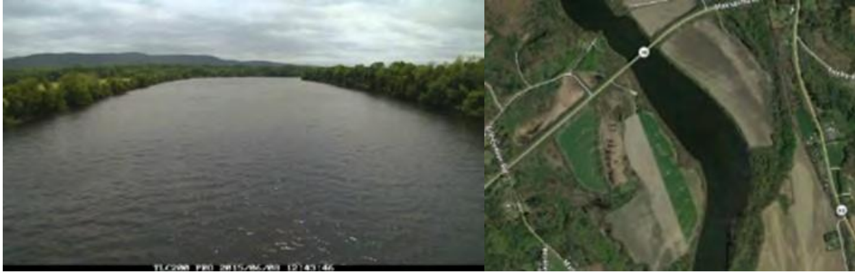
Figure 4.2.8.4-4: Rt. 10 Bridge Site CAM2 View and Aerial View (Google)
