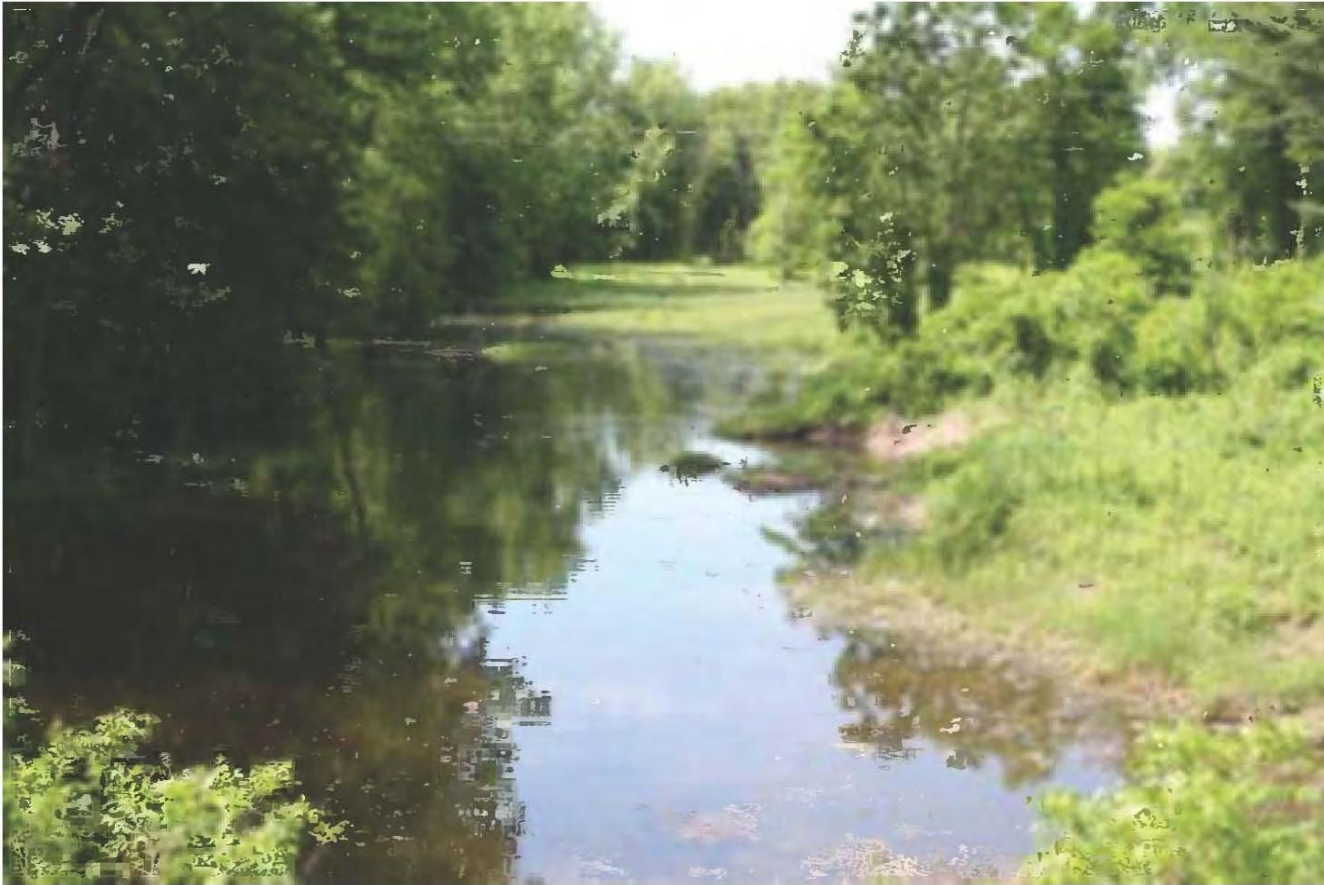
Figure 2.3.2-7 Abandoned avulsion channel behind Schell Bridge (d) (Field, 2007)
