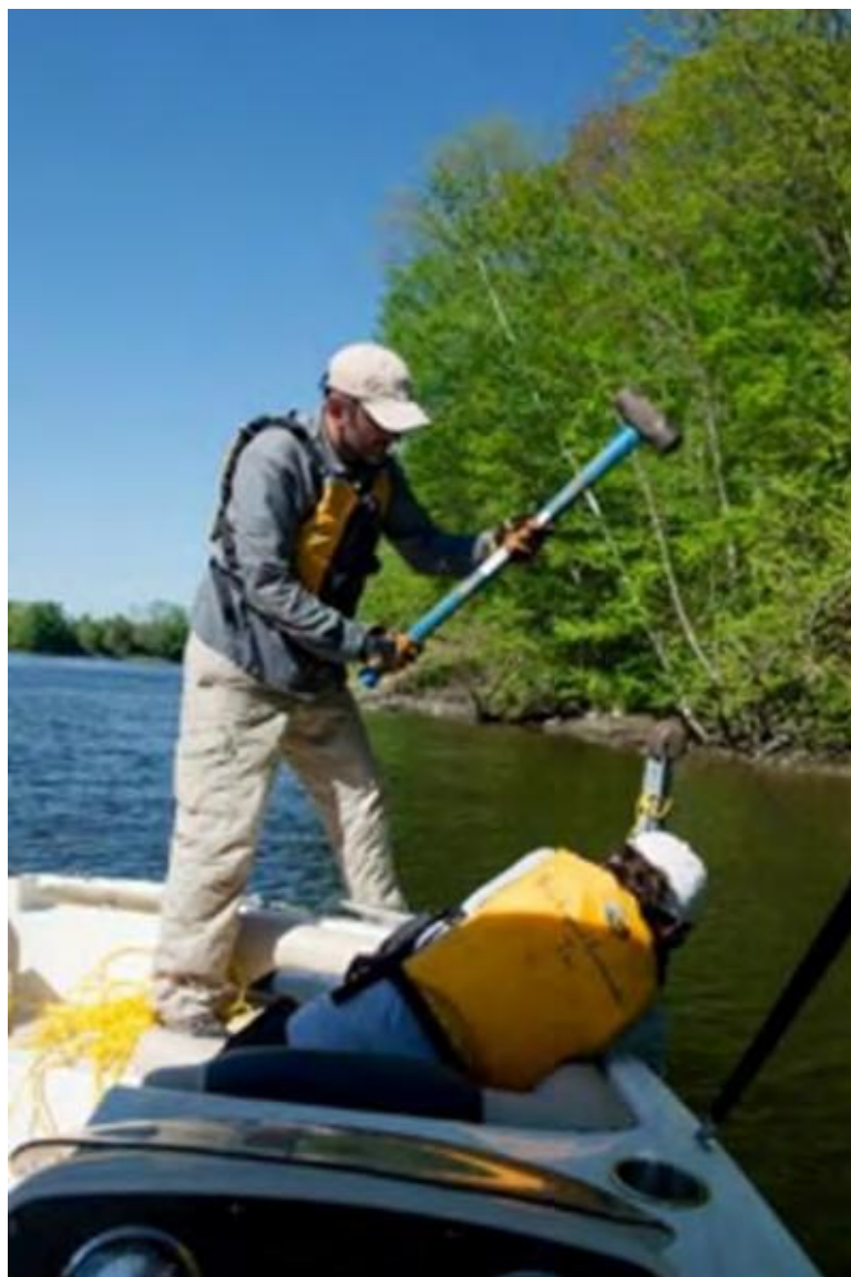
Figure 4.2.8.2-9: Installation of the T-posts
