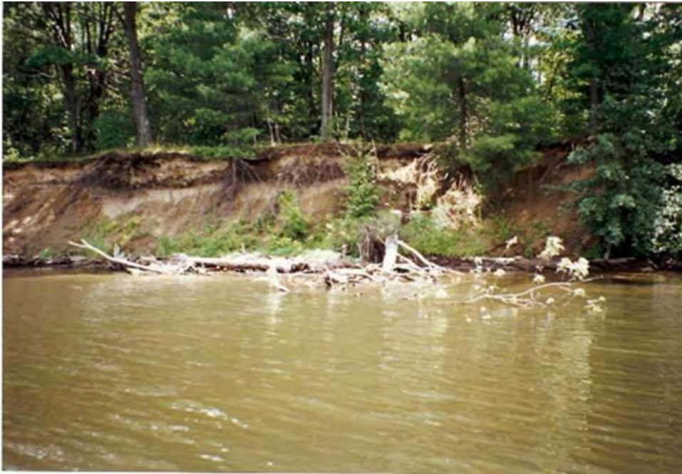
Figure 2.5-7: Vernon Impoundment – Location I (1997)
