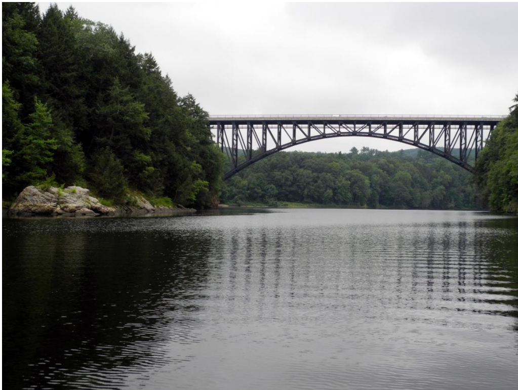
Figure 3.3.9.1.2-2: French King Bridge over Turners Falls Impoundment
