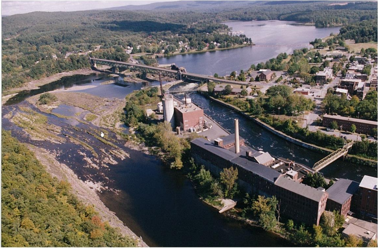
Figure 3.3.9.1.2-3: Aerial View of Turners Falls Dam Area, Looking Upstream
