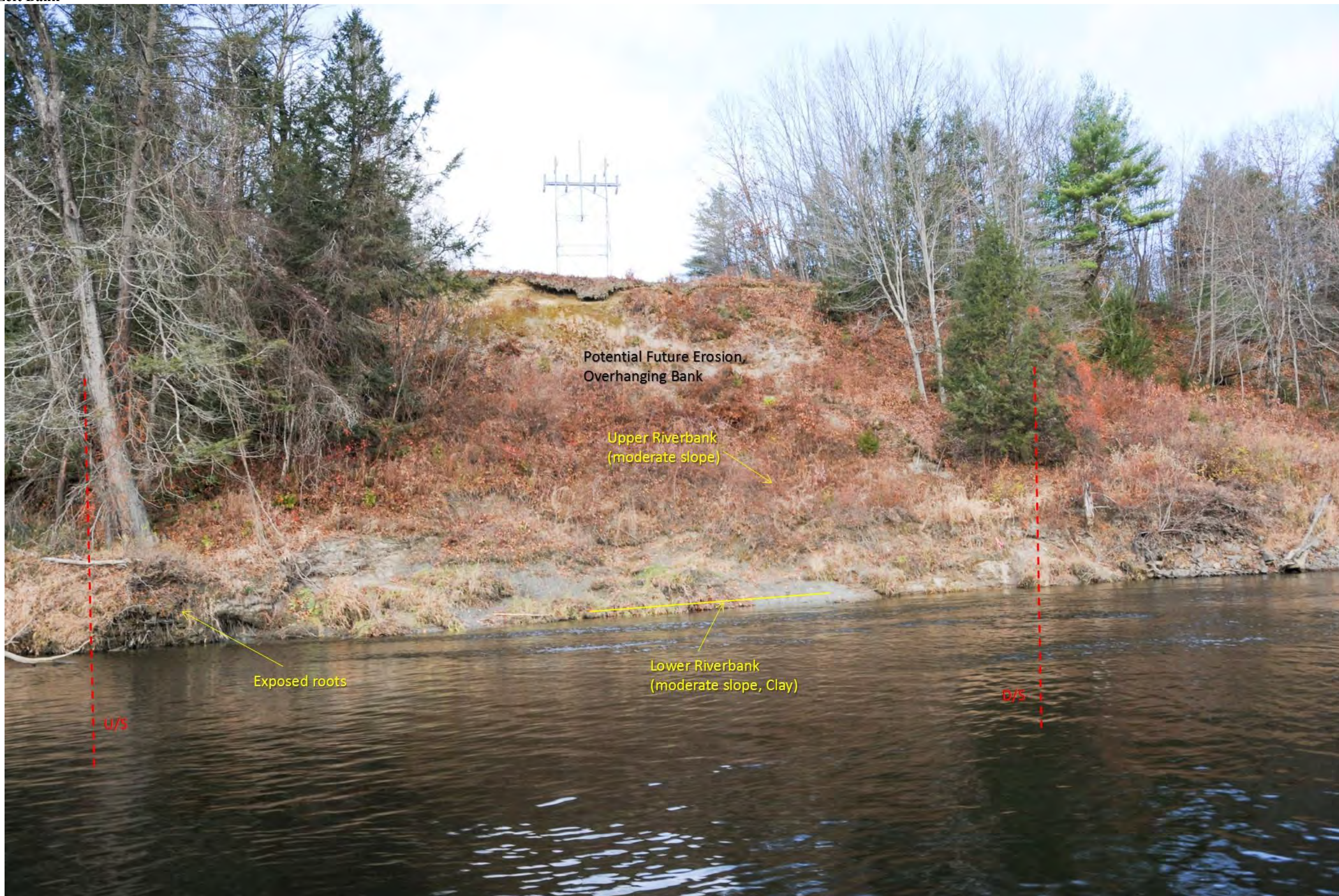
Photo ID 1425 (photo covers segment)
