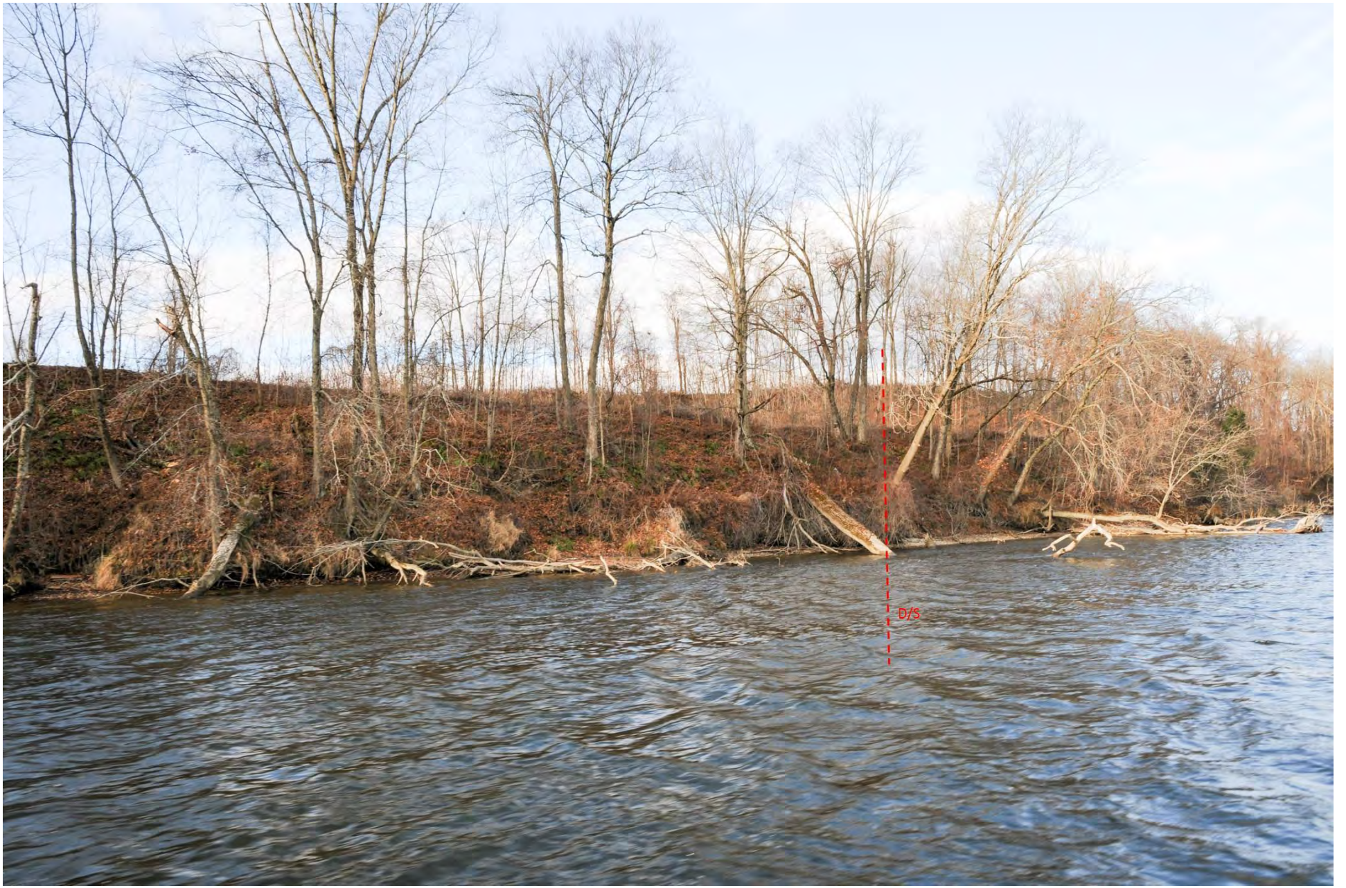
Photo ID 1239 (D/S, right of line)
