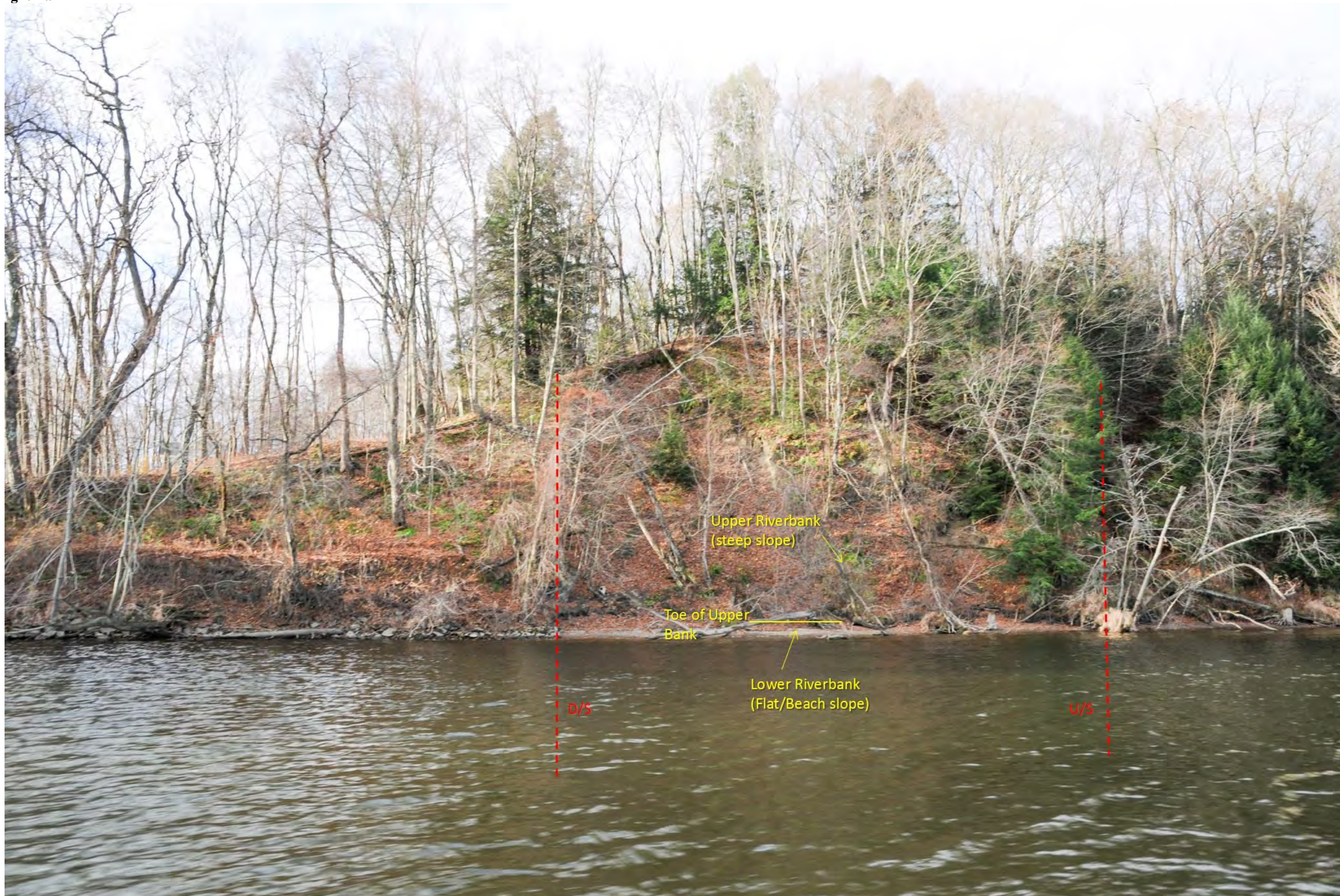
Photo ID 1114 (photo covers segment)
