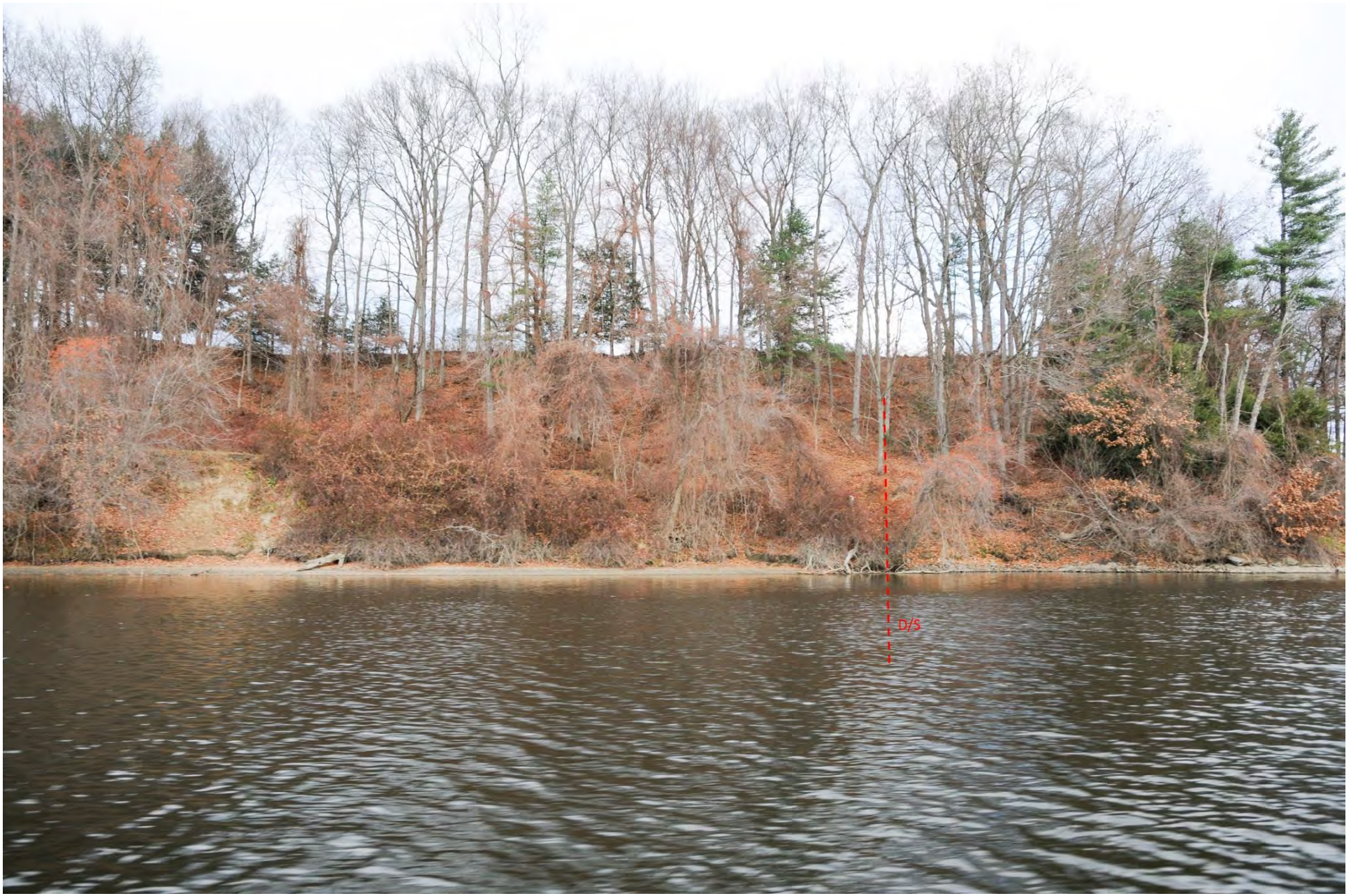
Photo ID 1003 (D/S, right of line)
