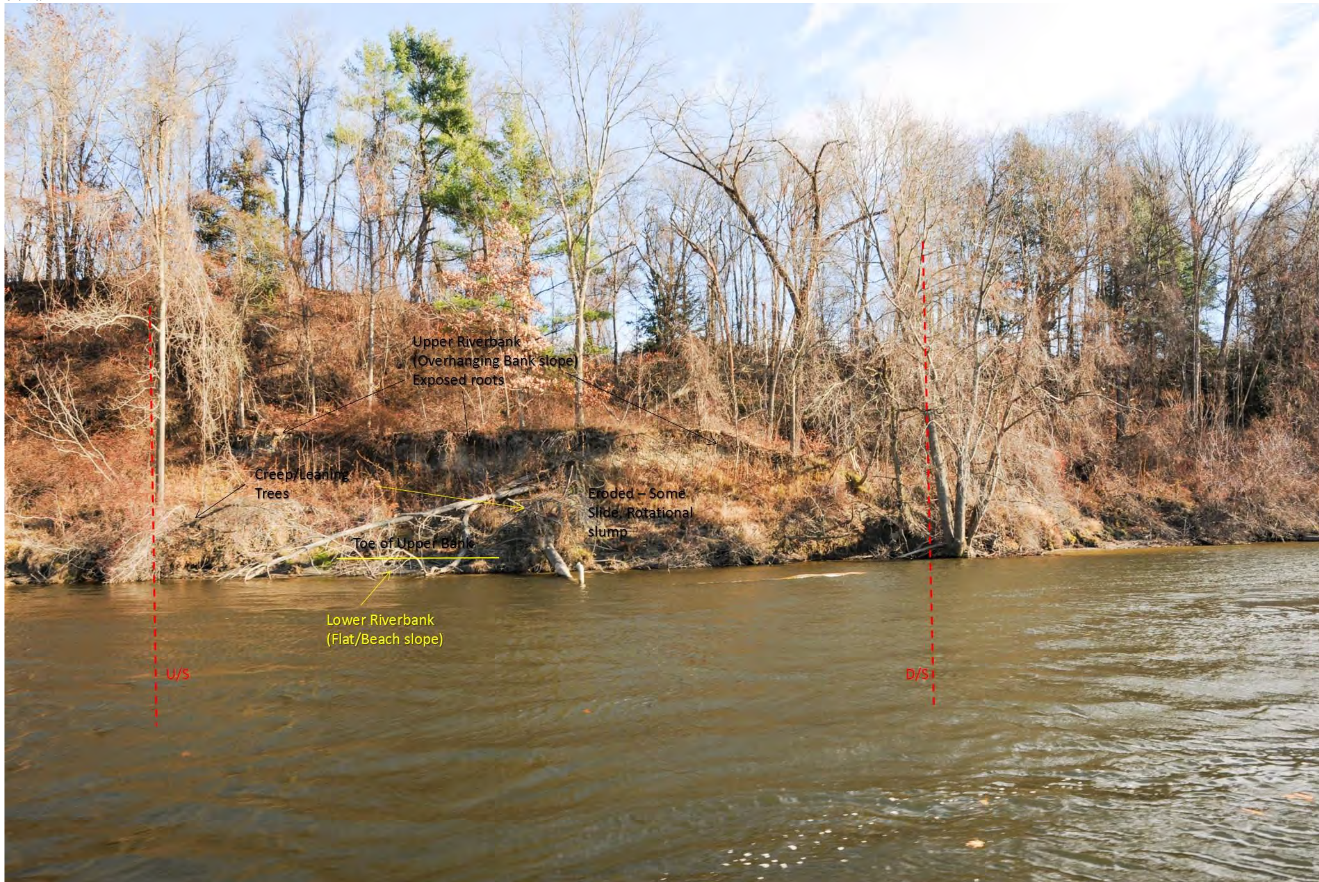
Photo ID 1670 (photo covers segment)
