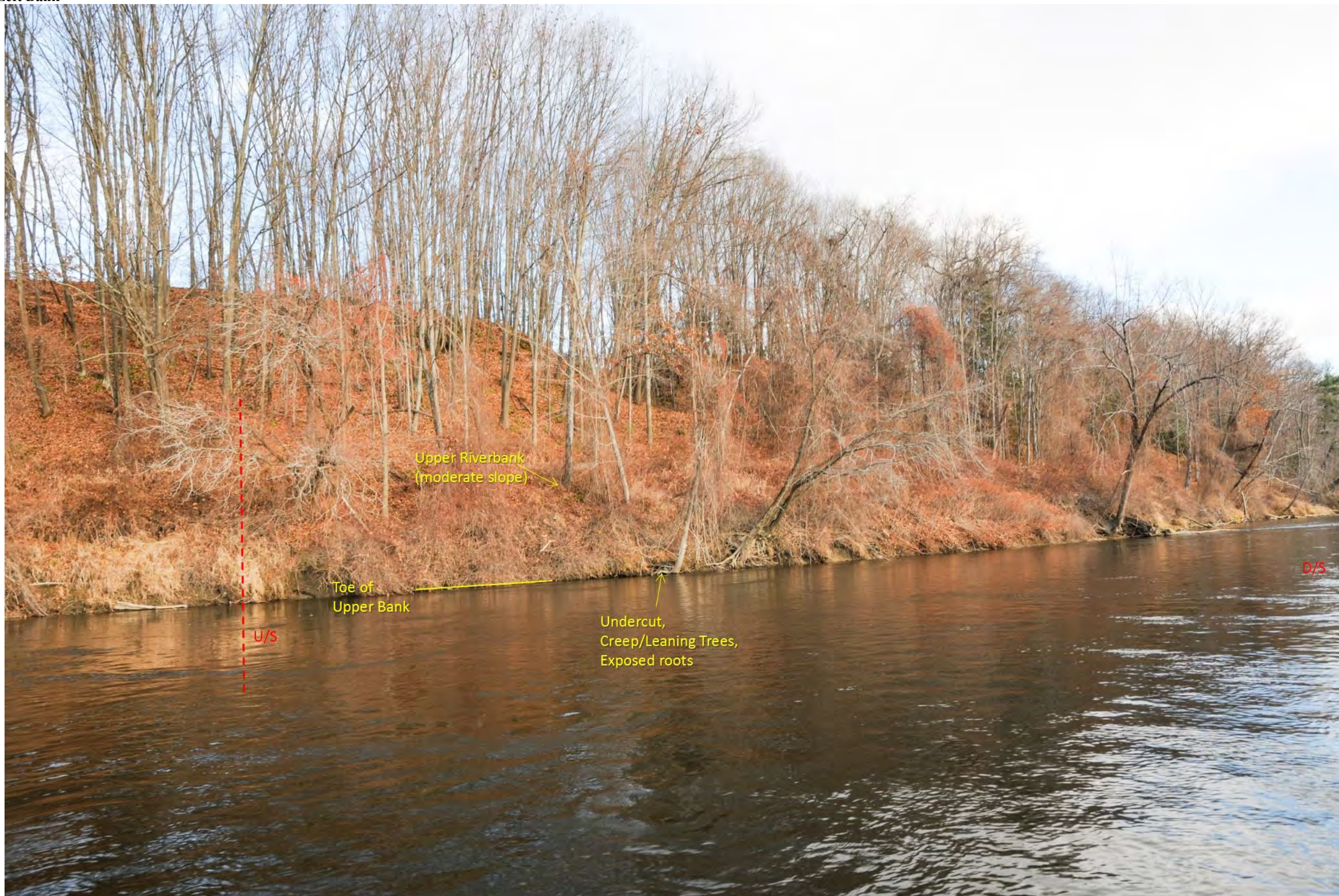
Photo ID 1447 (photo covers segment)
