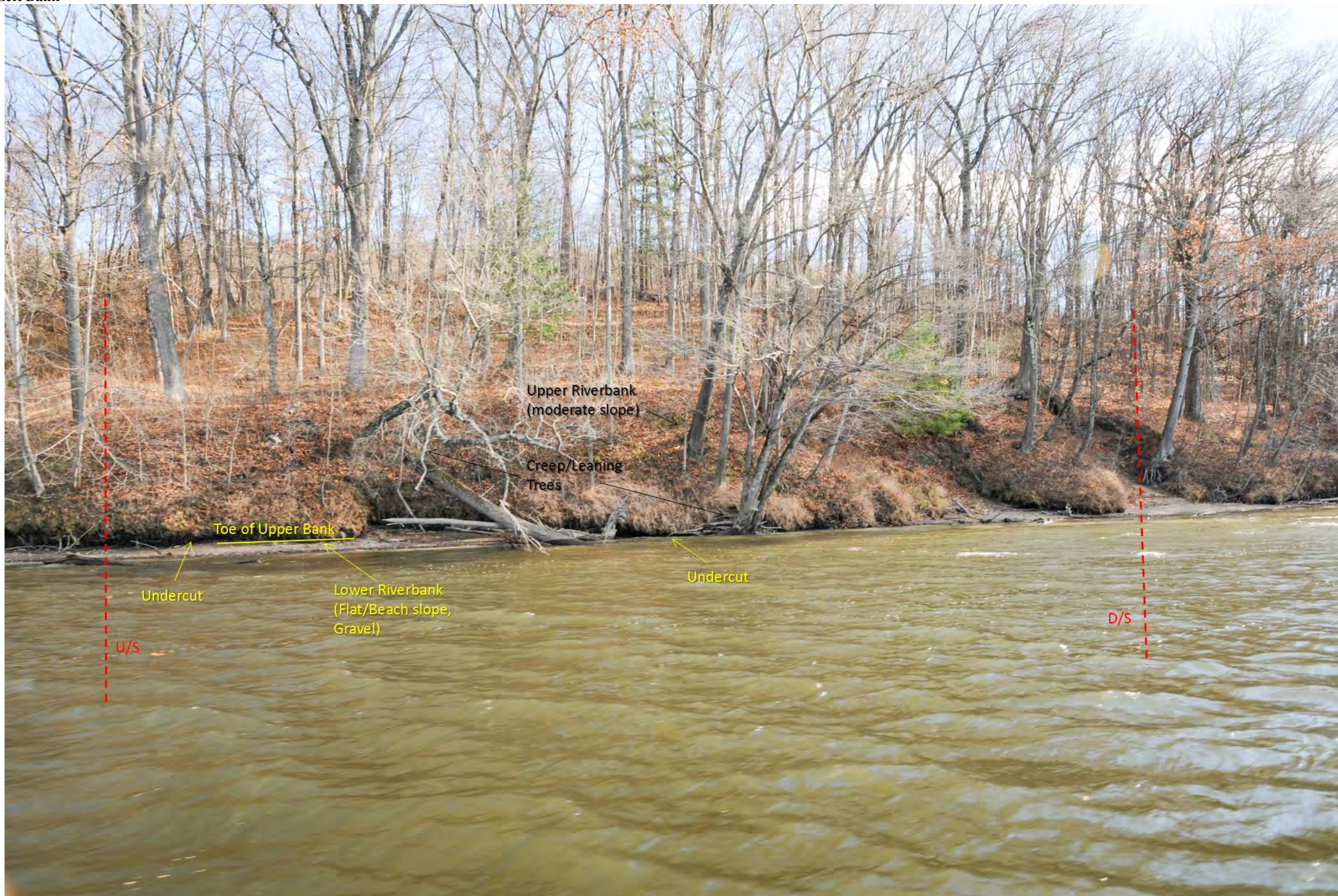
Photo ID 1605 (photo covers segment)
