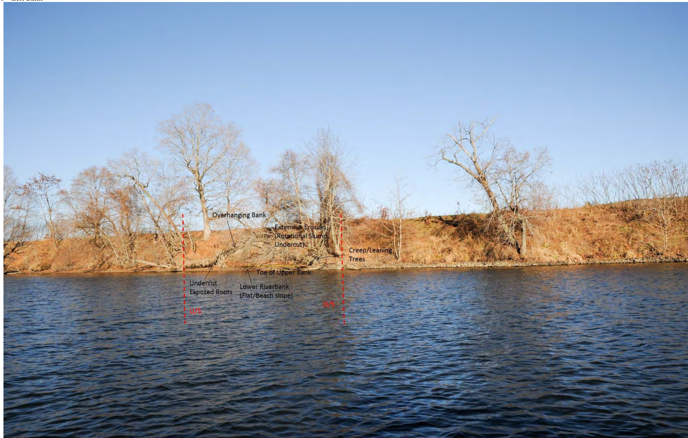
Photo ID 613 (photo covers segment)
