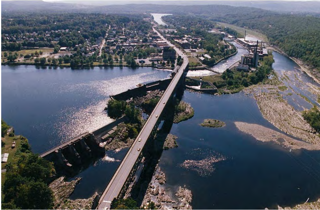
Figure 2.1.5a – Turners Falls Dam, Bypass Channel, and Power Canal (looking downstream)
