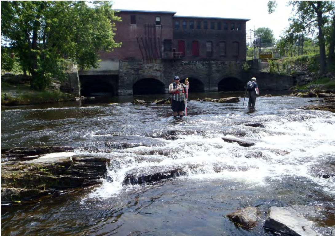
Figure 2.1.5b – View of Station No. 1 from Bypass Channel
