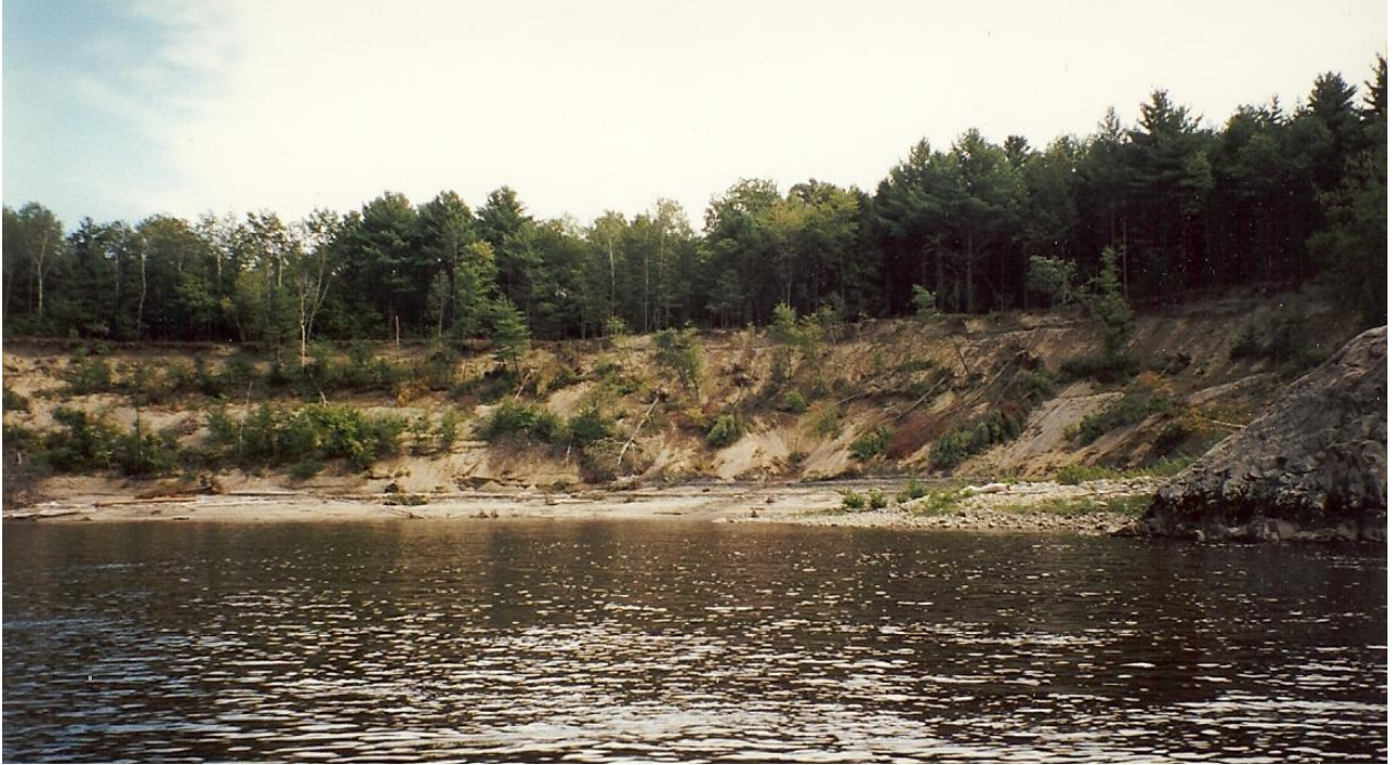
1996 – Eddy-induced erosion downstream of Vernon Dam
