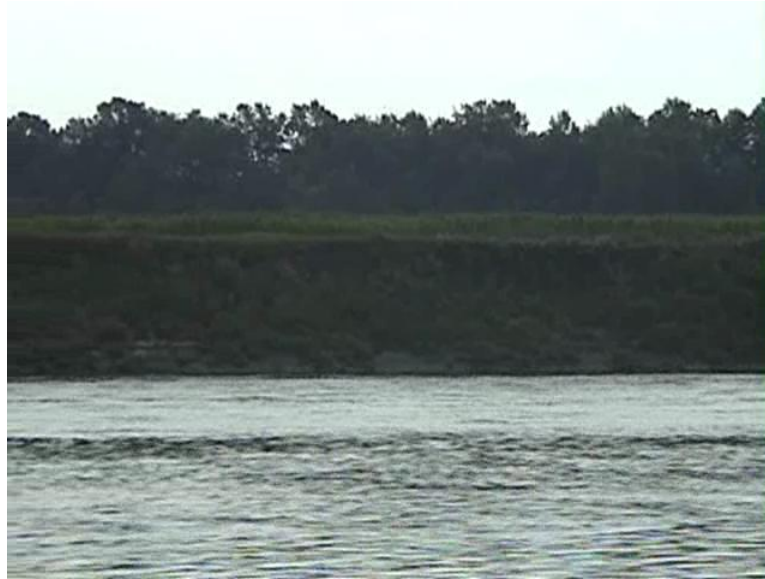
Right Bank near downstream end of Stebbin's Island - 1998
