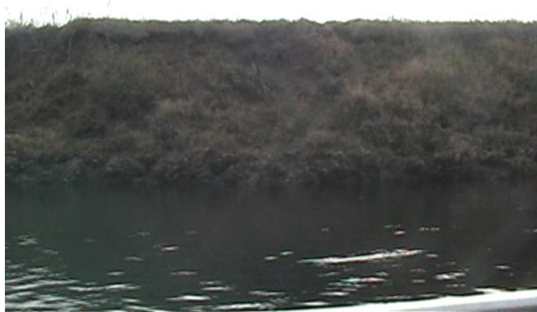
Right Bank near downstream end of Stebbin's Island - 2008
