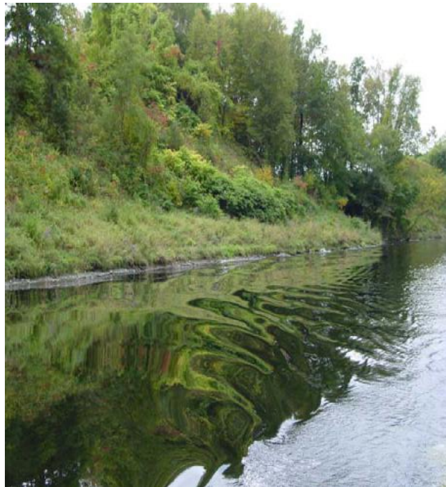
Site 6 – Skalski, 2008 (from Maintenance Inspection Report)
