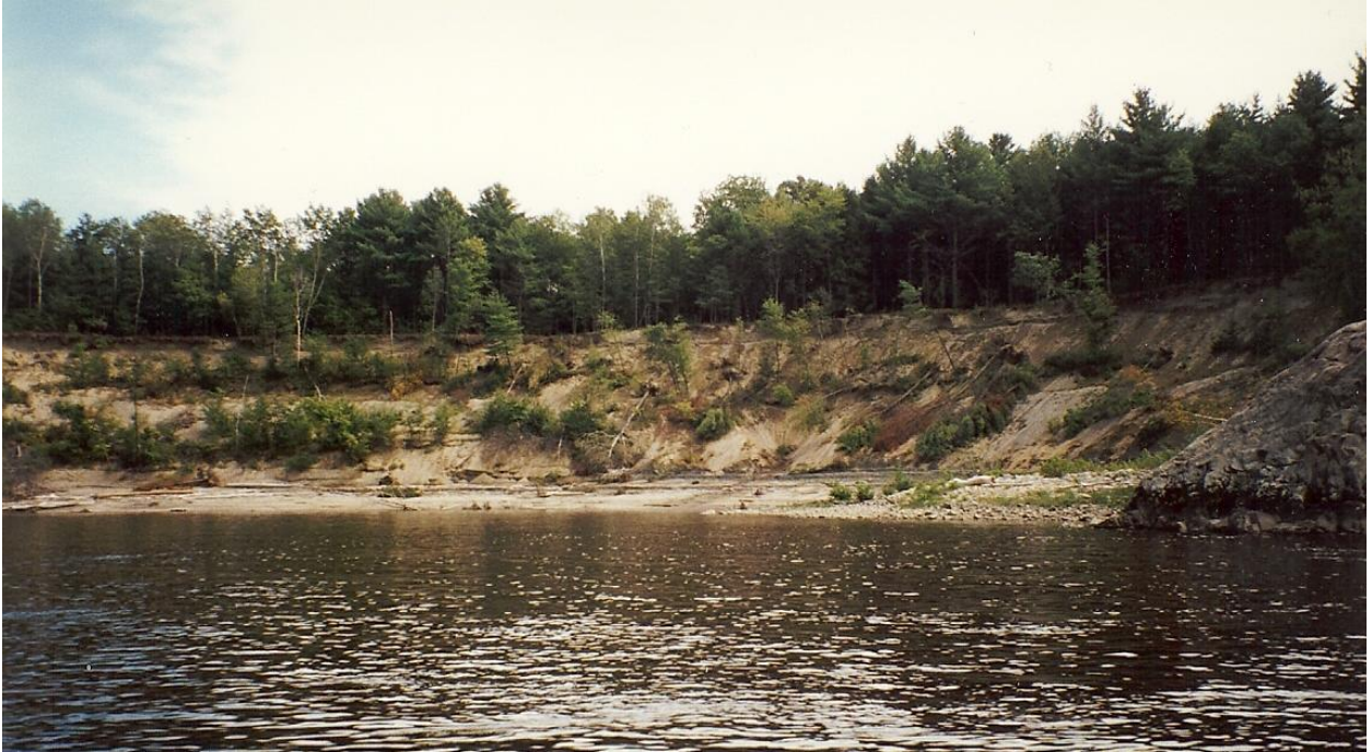
1996 – Eddy-induced erosion downstream of Vernon Dam
