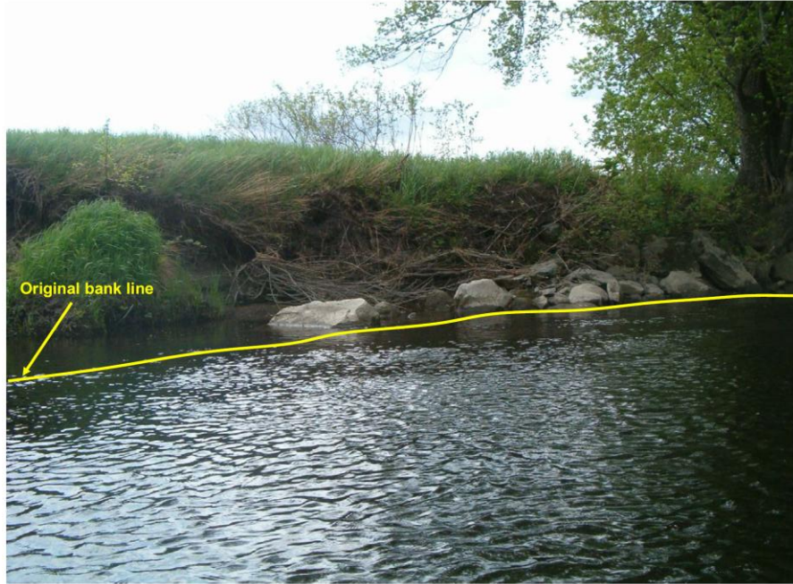
Figure 5. Erosion in channelized reach (after Field, 2004)
