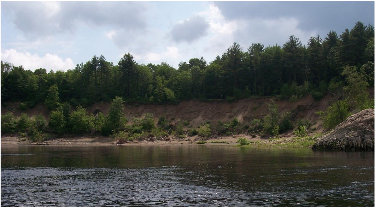
2008 – Eddy-induced erosion downstream of Vernon Dam
