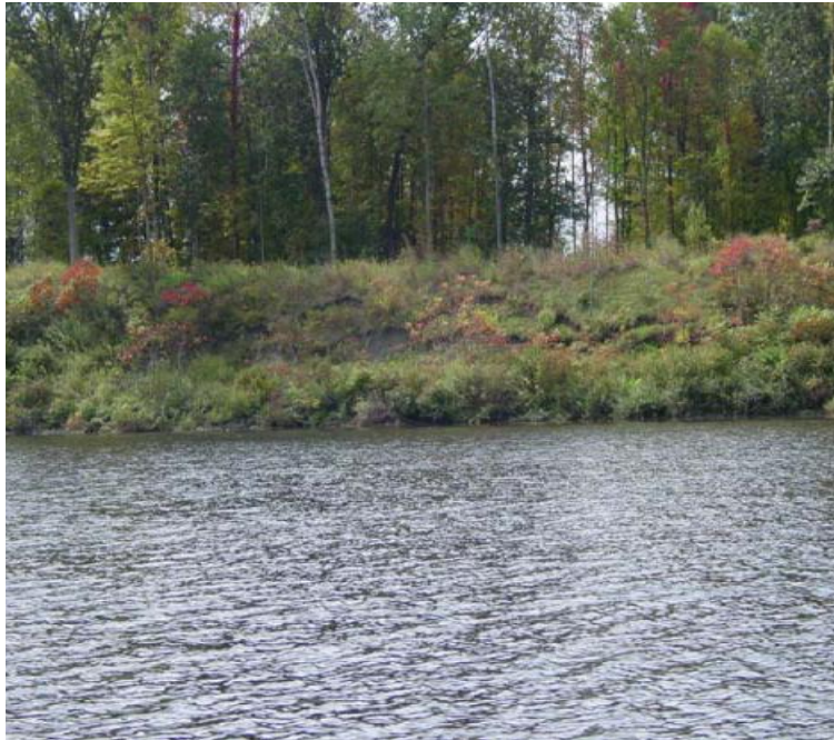
Site 4 – Urgiel (upstream), 2008 (from Maintenance Inspection Report)
