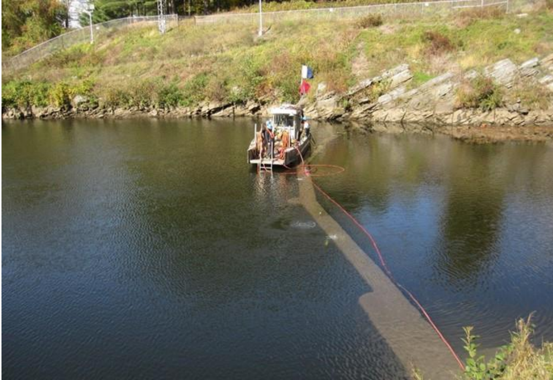
Figure 3.1.3-1. Concrete Wall at the Northfield Mountain Project Intake/Tailrace where Transducers were Installed to Monitor Juvenile Shad Entrainment
