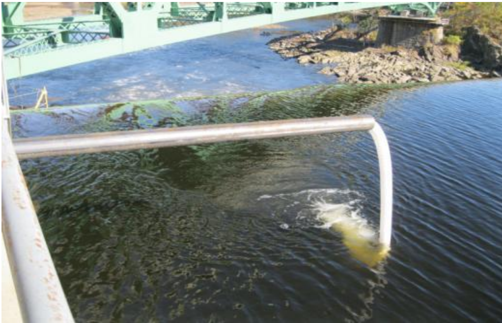
Figure 4-11 Metal pipe extension to release shad to the desired release point to ensure fish would pass over the Bascule Gates.
