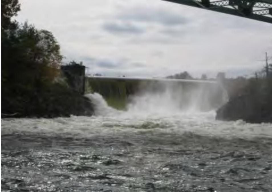
Figure 3-3 Downstream of Bascule Gate 4 at 5,000 cfs.
