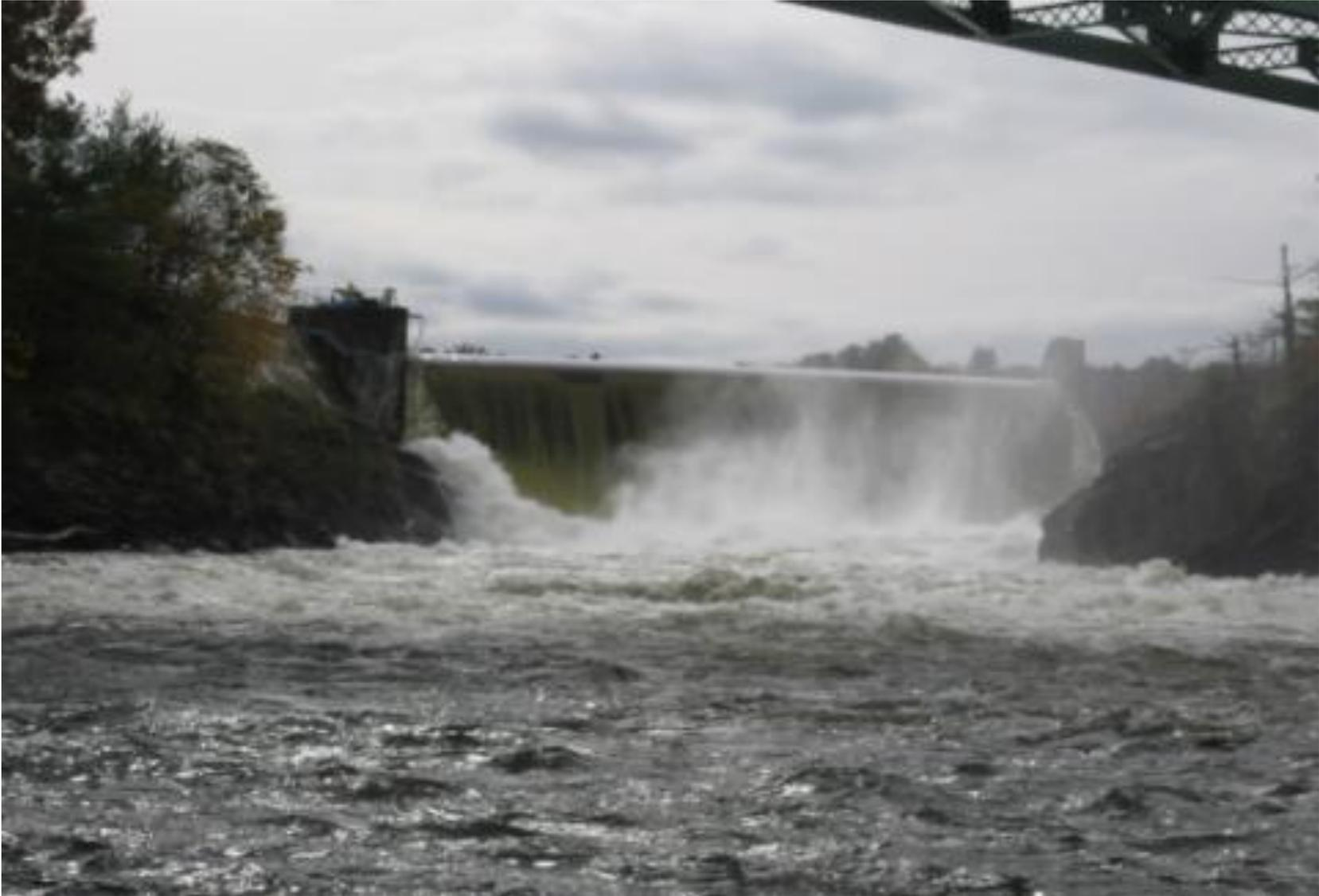
**Figure 2-3: Downstream of Bascule Gate 4 at 5,000 cfs.**
