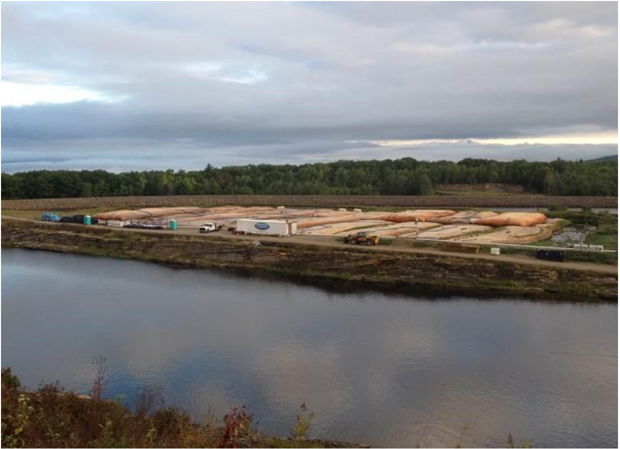
Figure 2.4-3 Geotube Dewatering System
