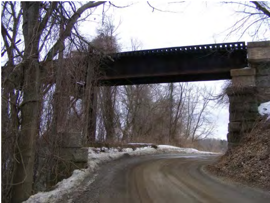
2014 View of Deck Girder over Caldwell Road (Source: TRC)
