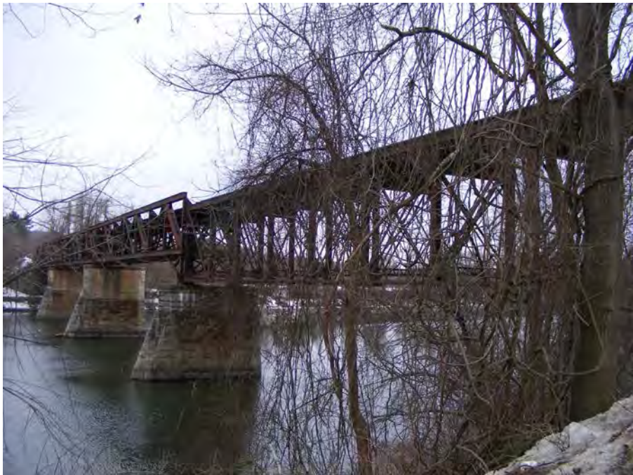
2014 View of Upstream Face (Warren Deck Truss: Left; Pratt Deck Truss: Right) (Source: TRC)
