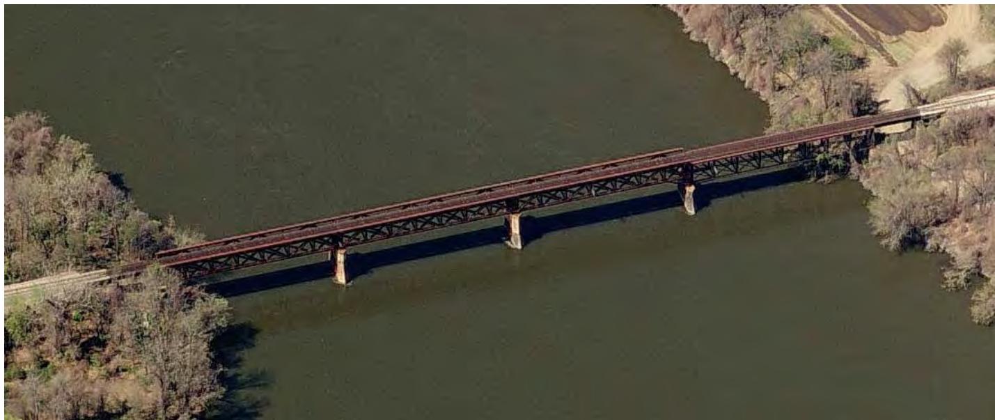
2008 Low-level oblique image of Vermont Central Bridge over Connecticut River (Left to Right: 1-span 1904 Deck Girder, 3-span 1936 Warren Deck Truss, 1-span 1904 Pratt Deck Truss, 1-span Deck Girder), (Source: MASSDOT GIS)
