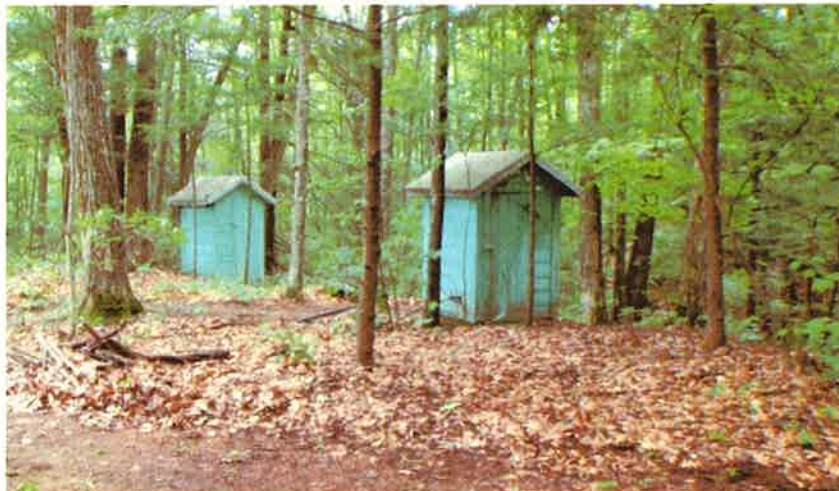
Camp 14E - two outbuildings, no longer in use, targeted for removal in 2010 report.
