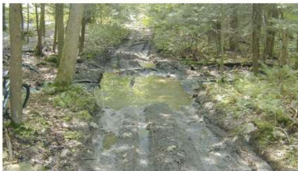
Photo of Problem Type: Mudholes
