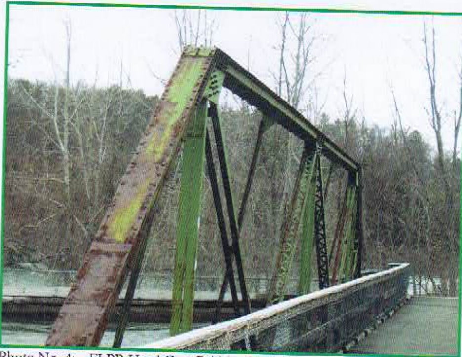
Photo No. 4: FLPR Head Gate Bridge - Typical configuration of truss Note condition of paint and areas of rust
