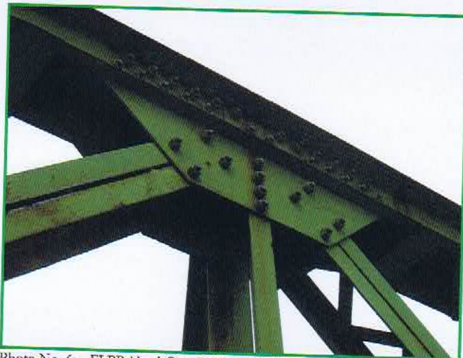
Photo No. 6: FLPR Head Gate Bridge - Typical connection along top chord
