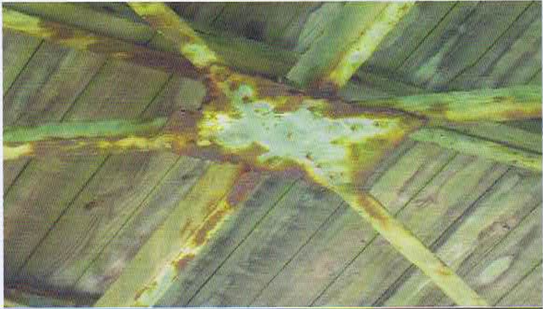
Gusset Connection Showing Corrosion & Material Loss
