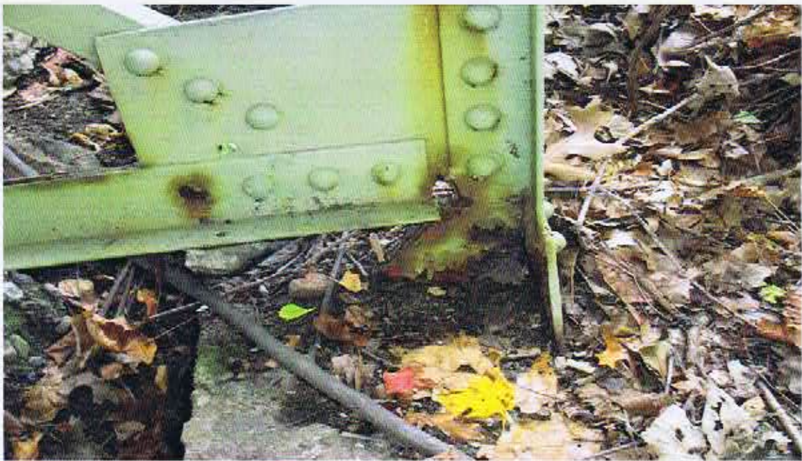
Base of Vertical Support Member Showing Rust Through
