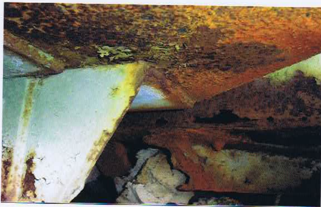
Corrosion Area below Bearing Support on Strathmore Side of Canal
