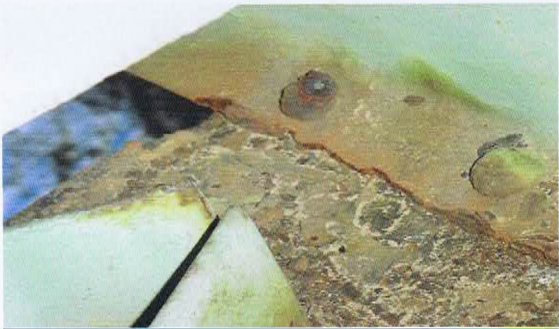
Gusset Connection Showing Corrosion & Material Loss
