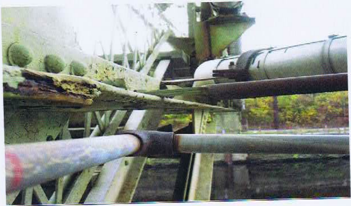
Main Support Chord Steel in Need of Repair at Connection Point
