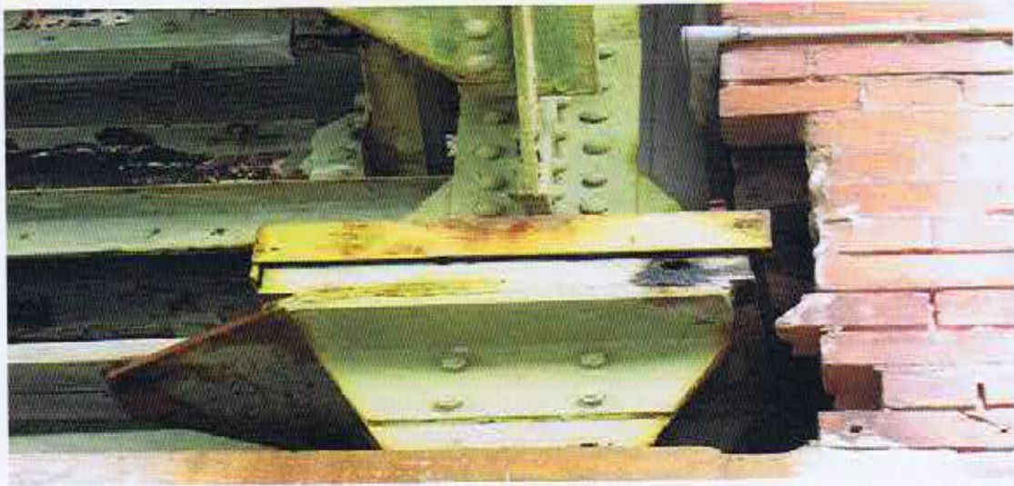
Bridge Bearing Support on Strathmore Side of Canal
