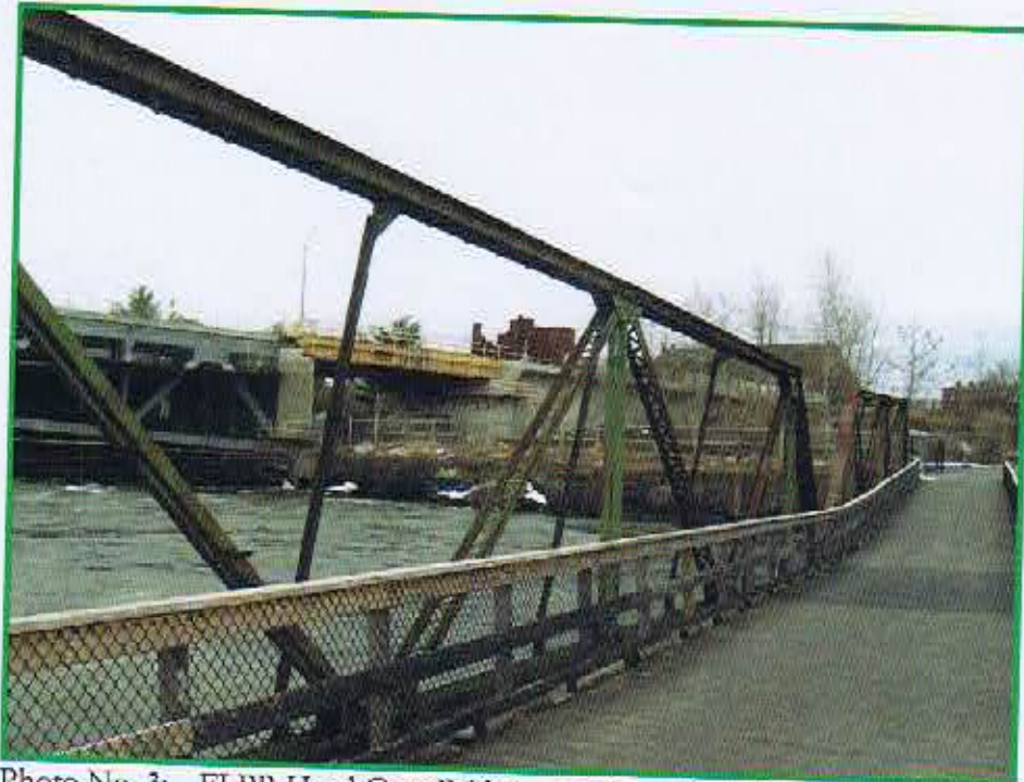
Photo No. 3: FLPR Head Gate Bridge – configuration of truss panels / bridge railing Facing northeast from western span
