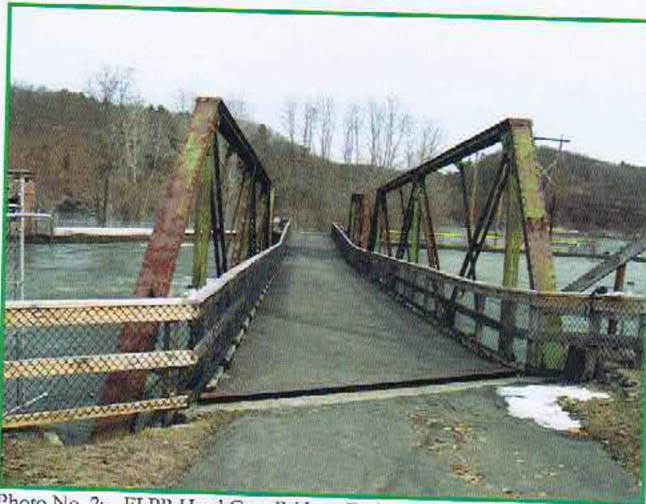
Photo No. 2: FLPR Head Gate Bridge - Facing west on east approach Note condition of paint / areas of rust / and open bridge joint
