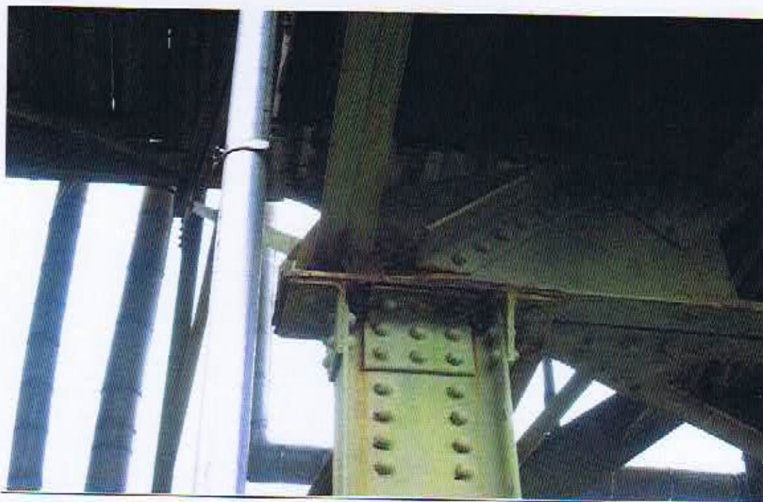
Corrosion Area at Top of Main Support Column on Canal Street Side of Canal
