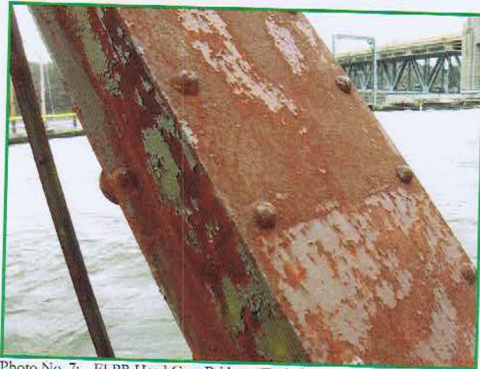
Photo No. 7: FLPR Head Gate Bridge – Typical area of surface rust Pitting with little to no section loss typical
