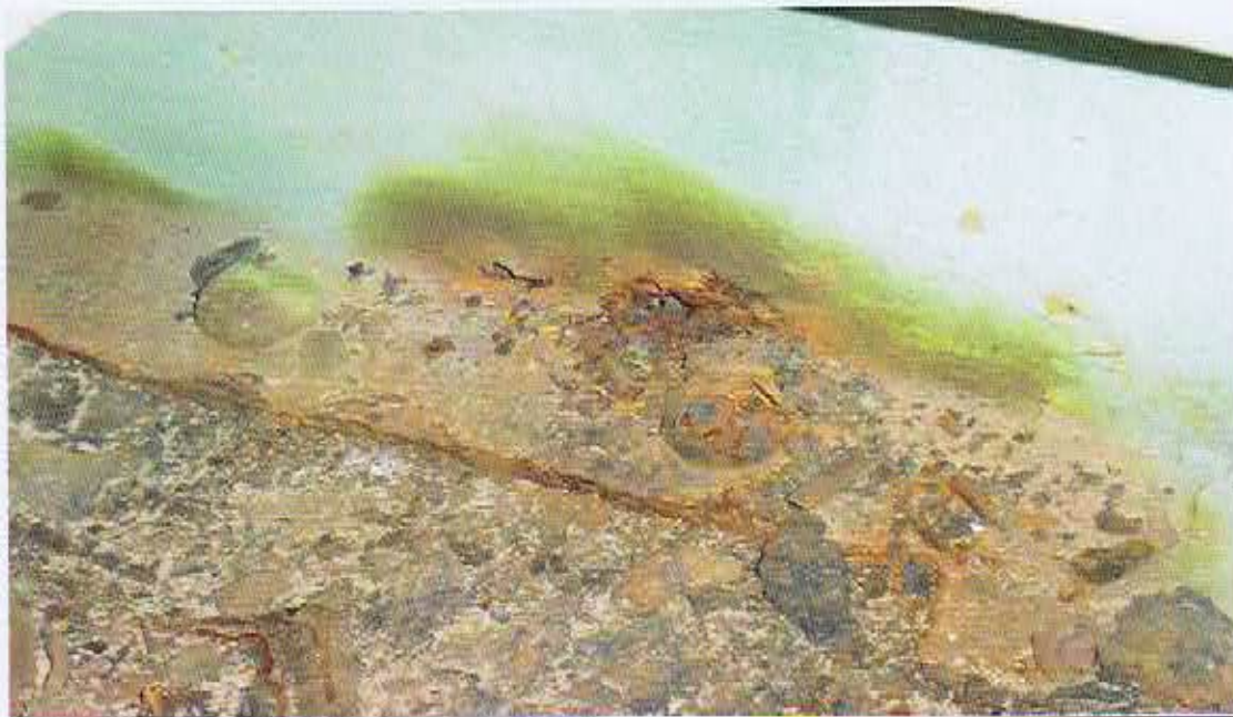
Gusset Connection Viewed from Above After Removing a 2 nd Plank
