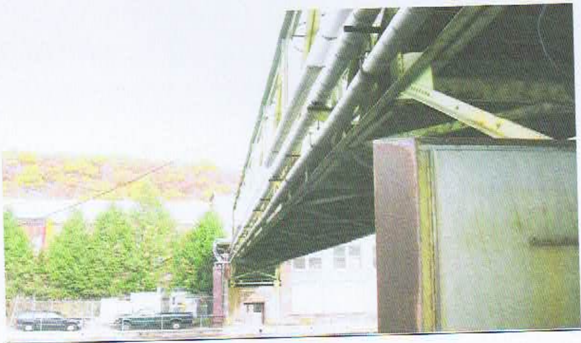
Main Support Chord Steel and Miscellaneous Utility Piping
