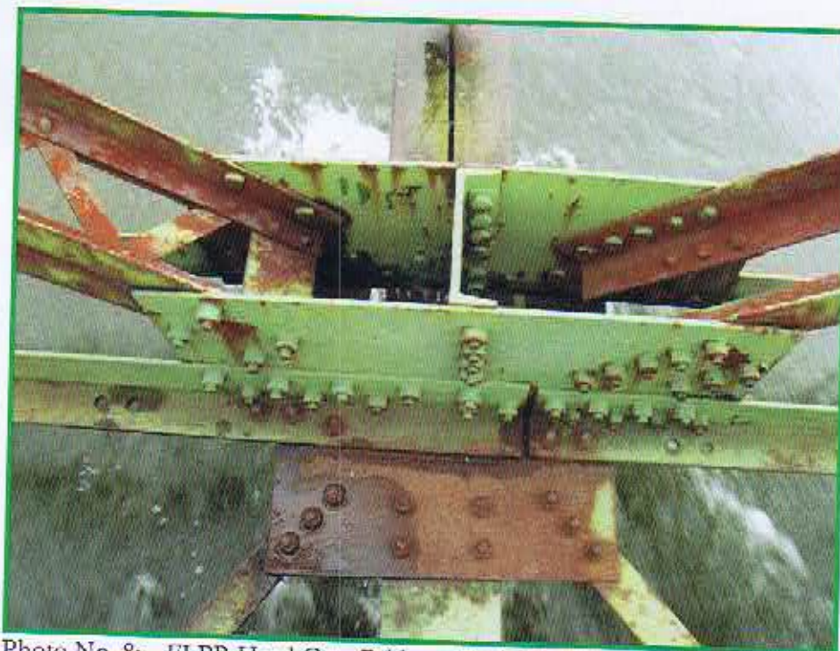
Photo No. 8: FLPR Head Gate Bridge – Typical bottom chord connection Note condition of paint and areas of rust
