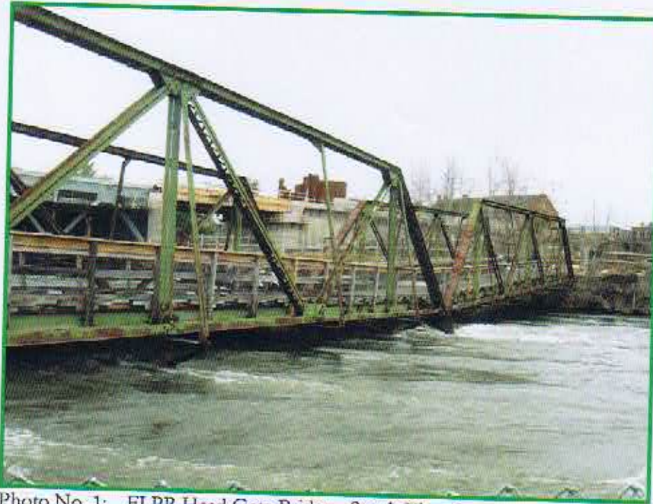
Photo No. 1: FLPR Head Gate Bridge - South Elevation Note condition of paint and areas of rust
