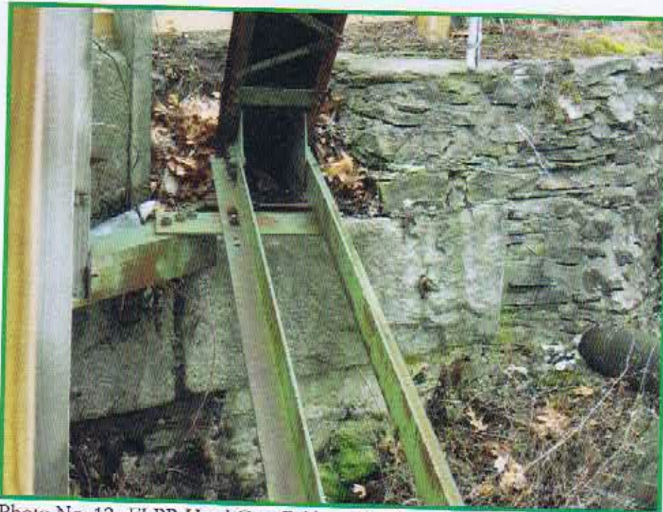
Photo No. 12: FLPR Head Gate Bridge – Southeast bearing of eastern span Note accumulation of debris on bearing seat
