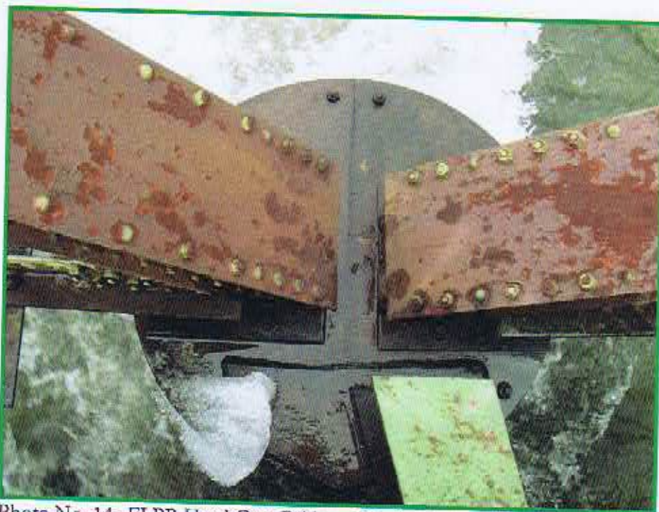
Photo No. 14: FLPR Head Gate Bridge – North caisson of steel pier bent Note condition of paint and areas of rust
