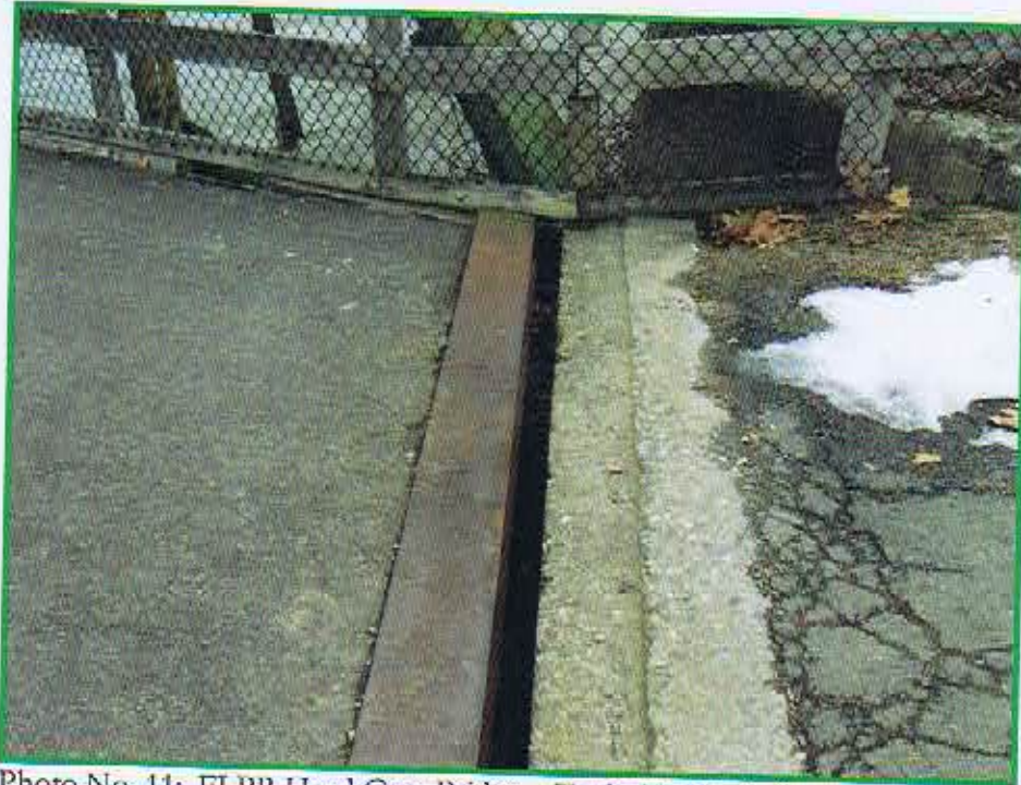
Photo No. 11: FLPR Head Gate Bridge – Typical bridge joint Note lack of actual bridge joint system
