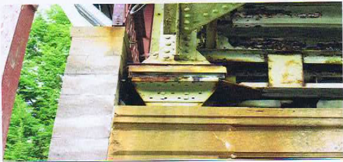
Bridge Bearing Support & Concrete Abutment on Strathmore Side of Canal
