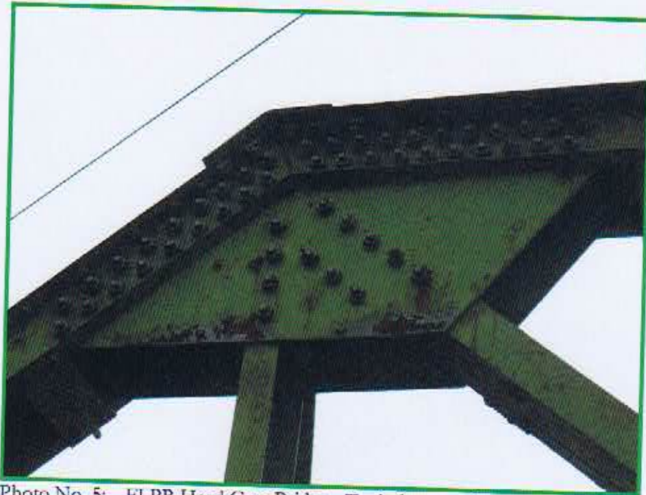
Photo No. 5: FLPR Head Gate Bridge - Typical connection at end of top chord
