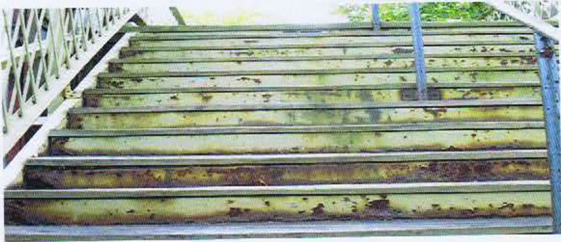
Front View of Stairway Showing Corrosion
