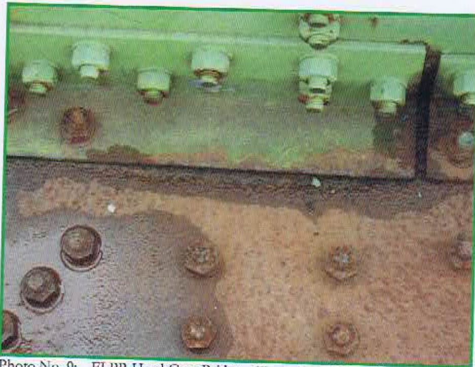
Photo No. 9: FLPR Head Gate Bridge – Typical condition of bottom chord connection Top surface of gusset plate - note area of section loss along leg of angle
