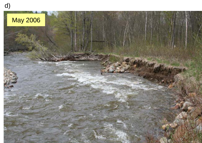
Figure 42: Time sequenced photographs showing collapse of bank armoring and continued erosion due to undermining on the South Branch of the Sandy River, ME.
