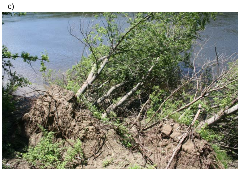
Figure 21: a) Vertical tension cracks lead to b) a topple blocks with tree attached and c) mounds of soil and roots at the base of the bank.
