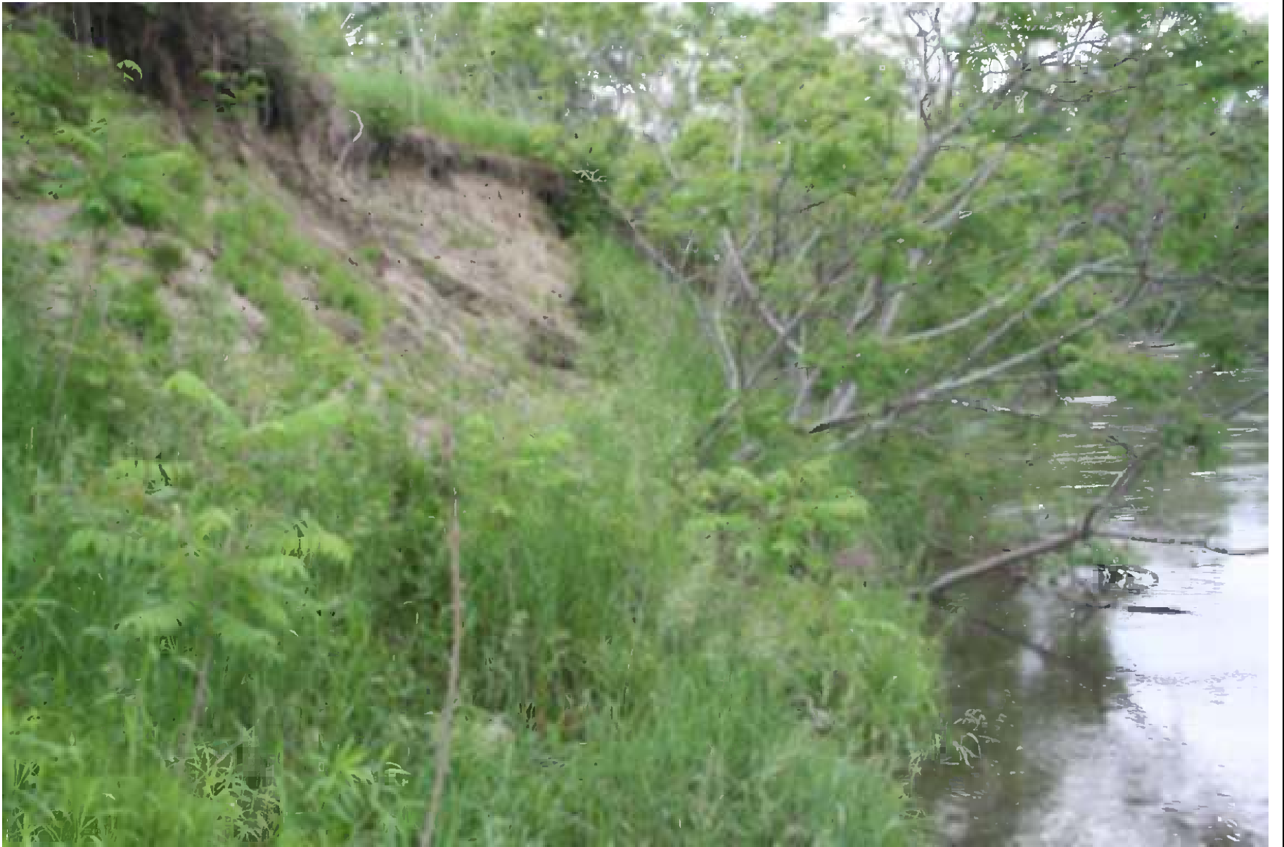
Figure 32: Active planar slip with vegetation growing on the surface.
