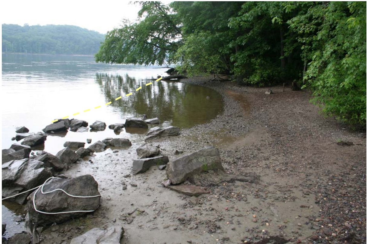
Figure 29: a) Bank recession continuing beyond riprap and b) failed section of riprap in Barton Cove (dashed line indicates former position of riprap).
