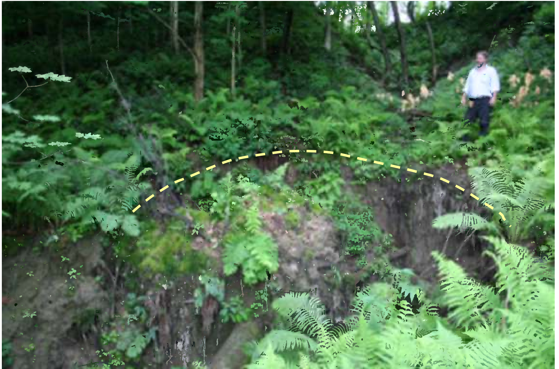
Figure 15: Active headcut on a small gully incised into a high bank downstream of Dry Brook. Note top of headcut is delineated by dashed yellow line.
