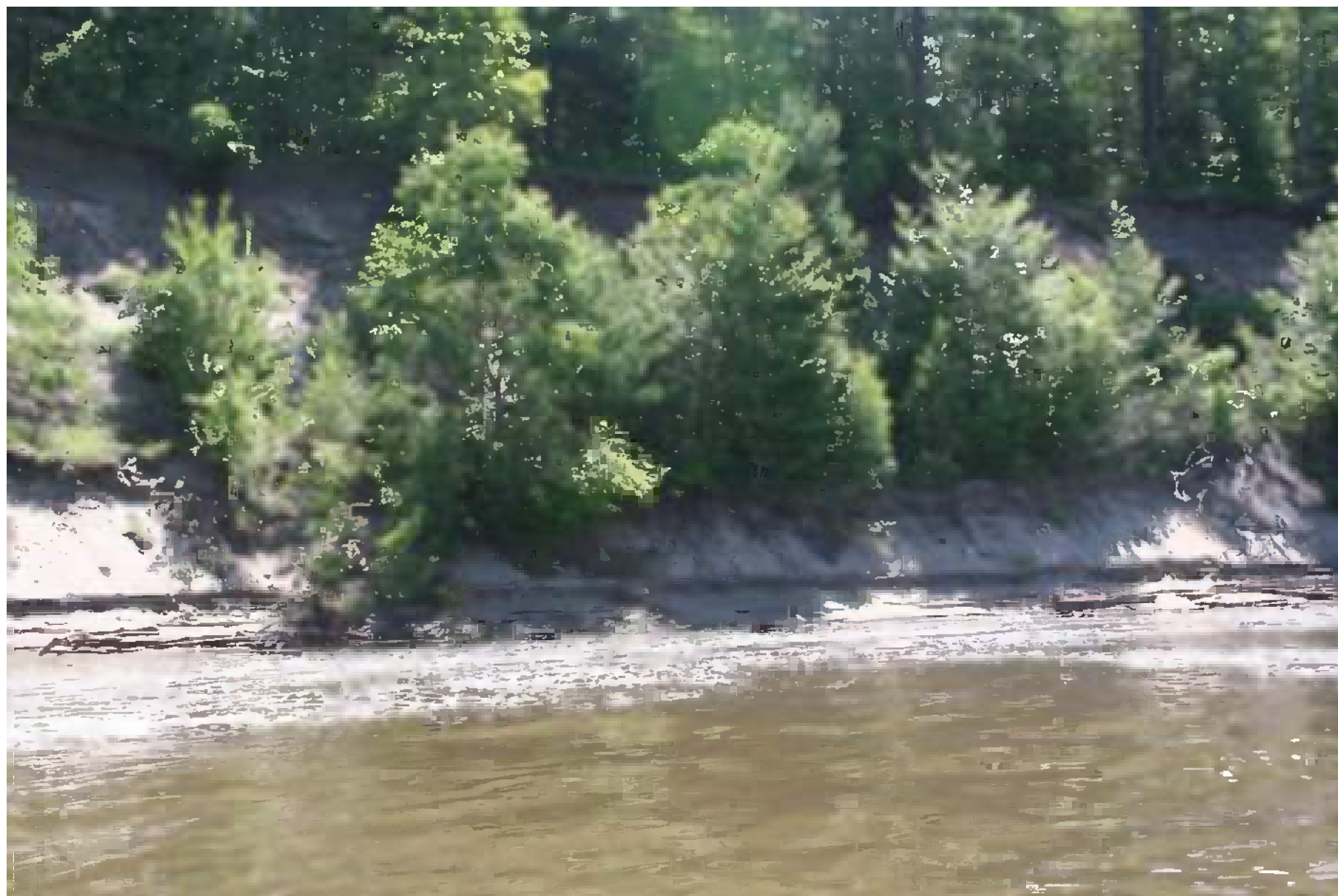
Figure 23: High eroding bank downstream of Vernon Dam showing trees still growing on bench at top of a slip block. Note colluvial apron formed from flow deposits below bench
