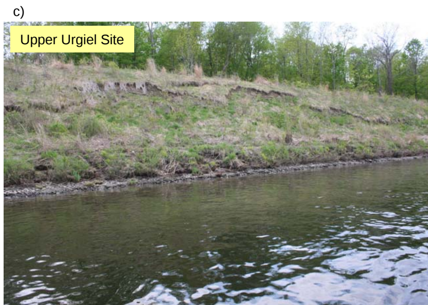
Figure 39: a) Coir logs removed by water currents, b) coir logs detached from bank by mass movements on upper slope, c) planar slips on upper slope resulting from removal of coir logs and notching at the base of the slope, and d) gully on the slope of a recently shaped bank.
