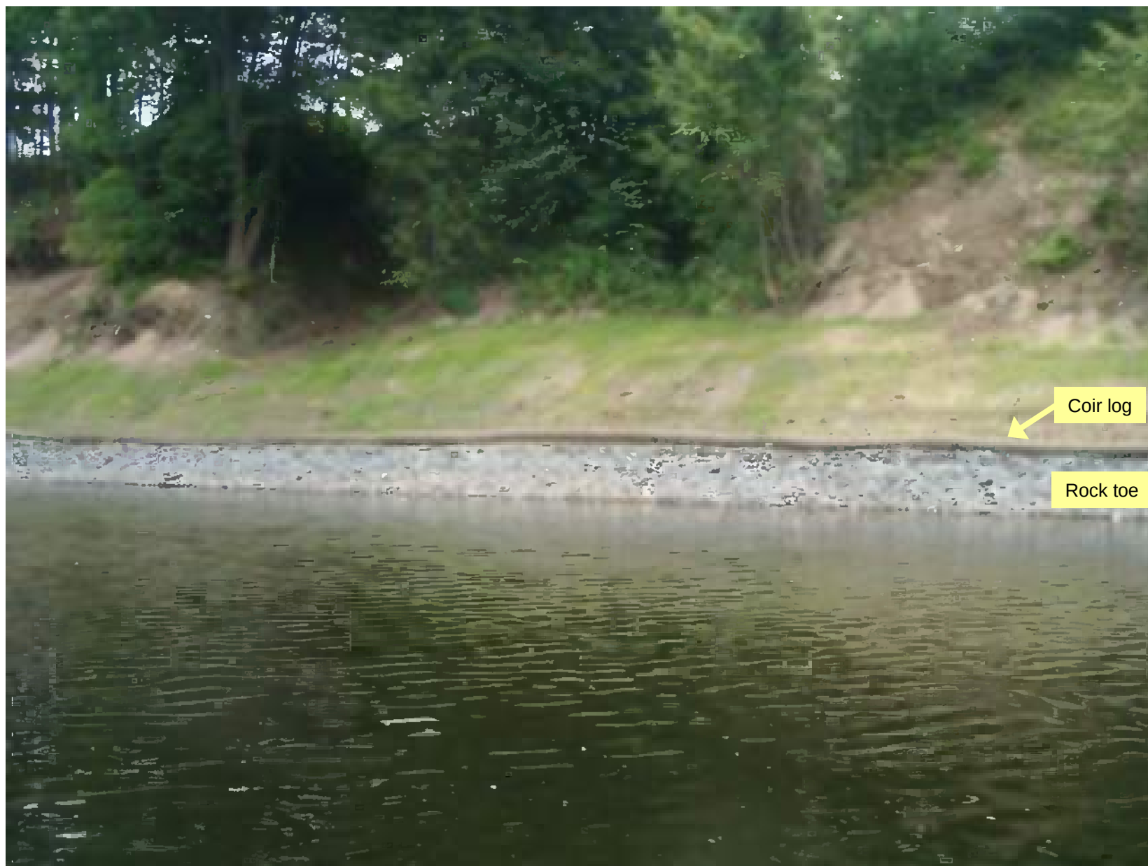
Figure 38: Bioengineering project (Skalski Site) with rock toe and coir log above.
