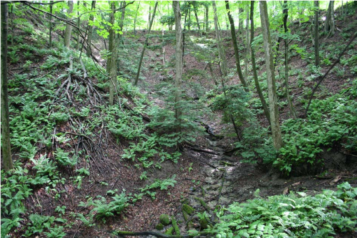
Figure 20: Gully formed by a) overland flow and b) groundwater seeps. Note berm in a) built to prevent additional overland flow from enlarging gully.
