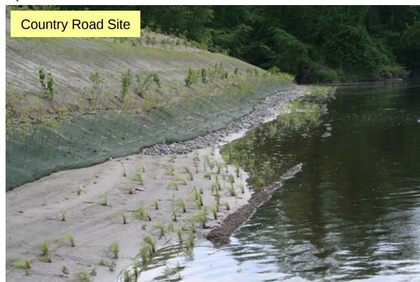
Figure 41: a) Vegetating bank face protected by beach despite logs removed from beach, b) low bench created during construction, c) floodplain bench created during construction, and d) coir logs placed under the water surface to encourage beach development.
