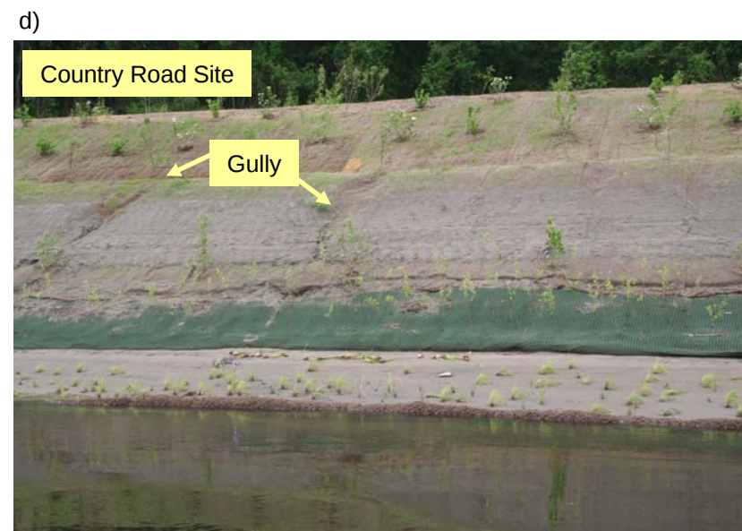
Figure 39: a) Coir logs removed by water currents, b) coir logs detached from bank by mass movements on upper slope, c) planar slips on upper slope resulting from removal of coir logs and notching at the base of the slope, and d) gully on the slope of a recently shaped bank.
